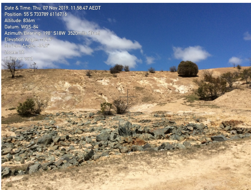
Figure 1 Vegetation failure and erosion on the western face of the waste rock emplacement
