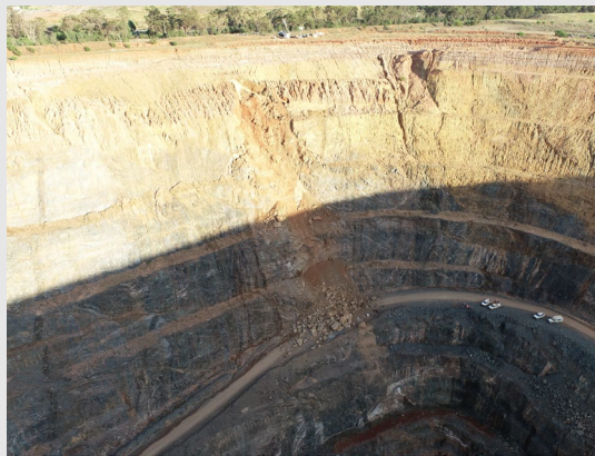
Ground or strata failure
