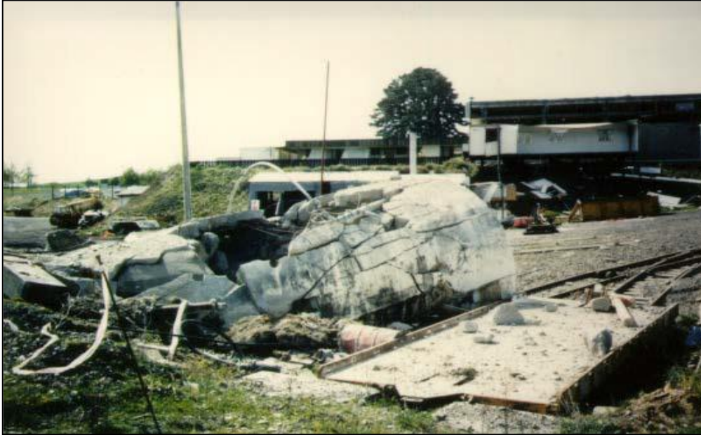
Figure 17: Blast damage to mine transport drift
