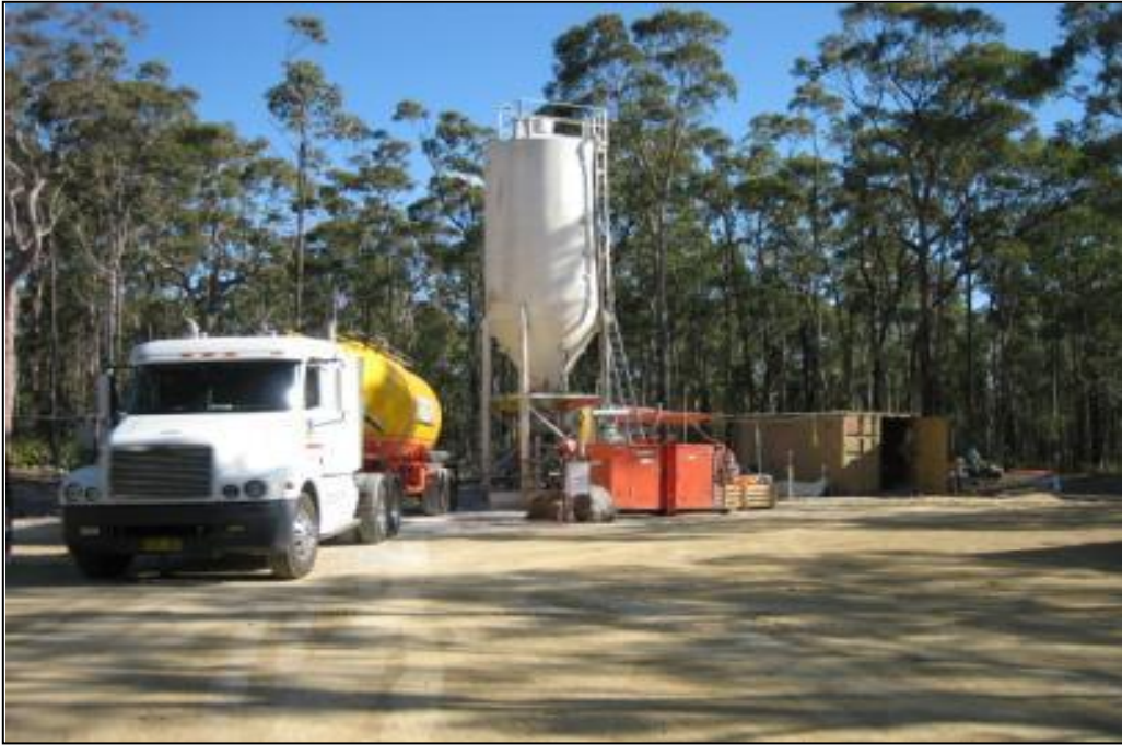
Figure 30: Surface plant for pumping fly ash seals
