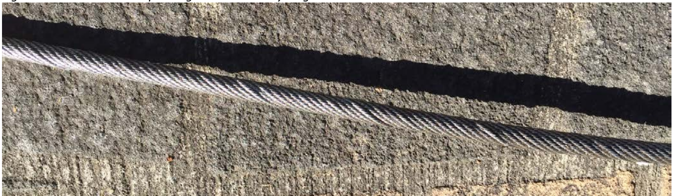
Figure 5 Proud wires corresponding to shortened lay length
