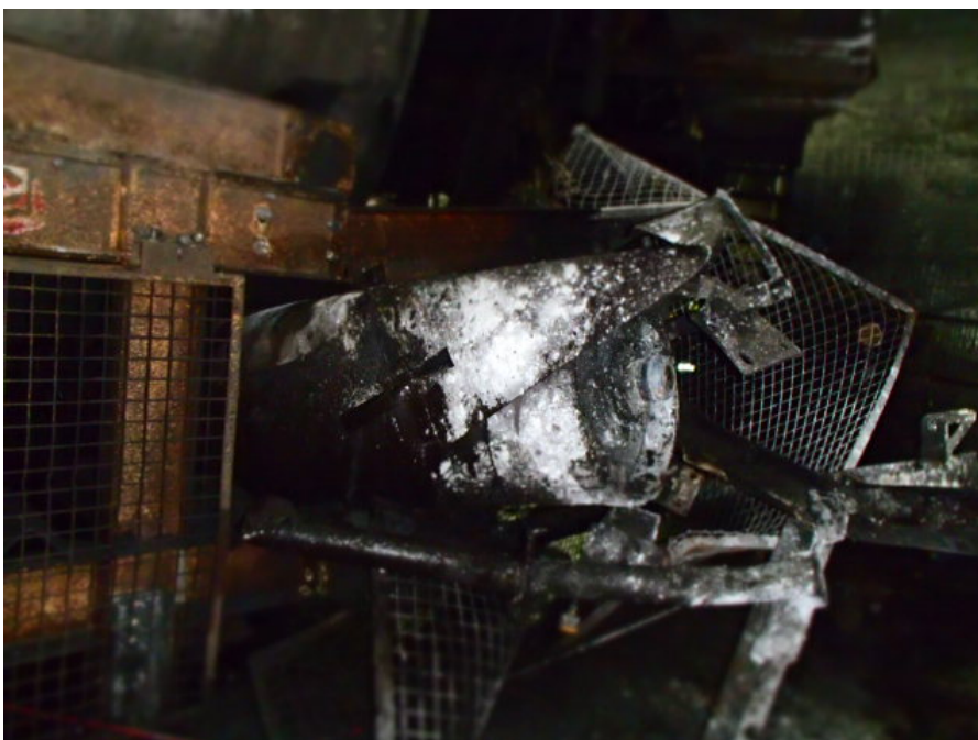
Figure 1 Failed pulley final location
