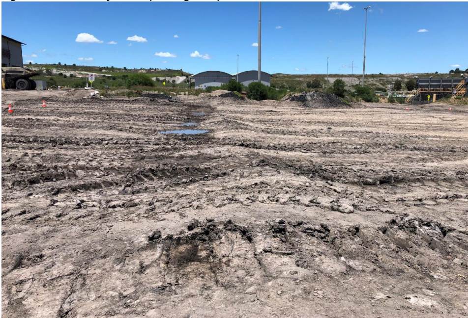
Figure 2 Condition of stable parking hump
