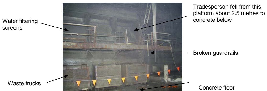
Photograph of fixed underground plant
