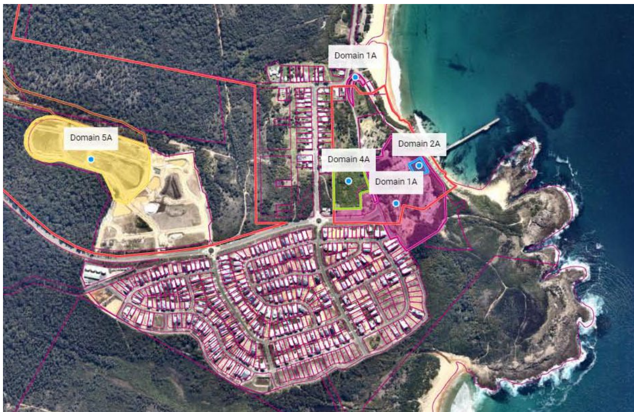
Figure 1: Mine closure domains (areas) associated with the former Catherine Hill Bay Coal Preparation Plant
