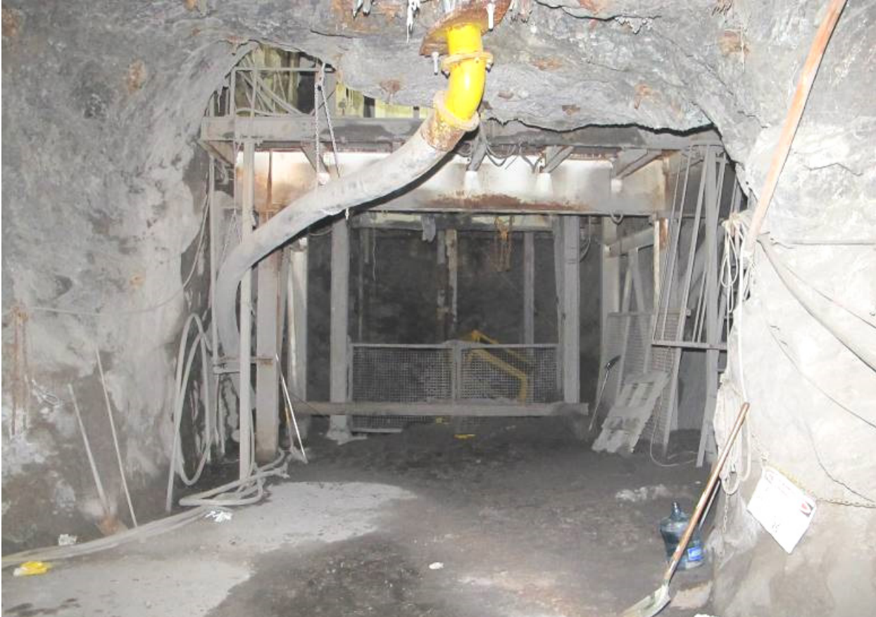
Figure 5: The 26 sub level access to the NBHC haulage shaft. This is the access into the base of the weigh flask above at the 26 level. Note the position of the horizontal steel RSJs and the closed steel mesh gate that formed the barriers across the front of the NBHC haulage shaft. 11
