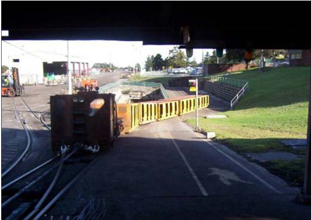
Figure 15 Drift haulage control and personnel cars (personnel transport system)
