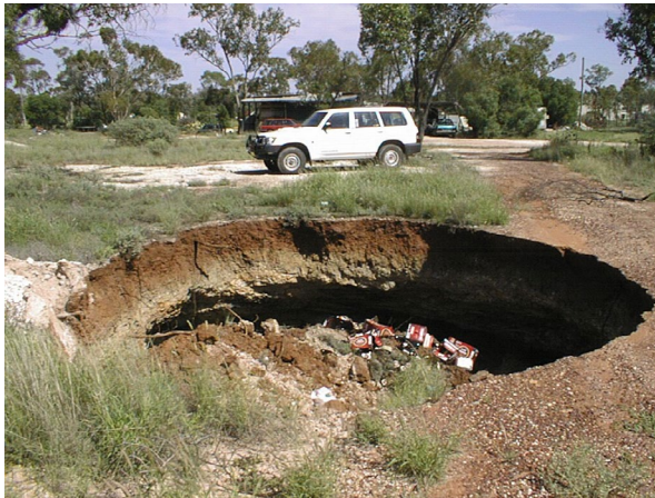
Figure 50 - Mine workings that subsidised due to inadequate primary support
