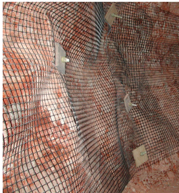
Figure 72 - Pillar support using plastic netting and fibreglass rock bolts
