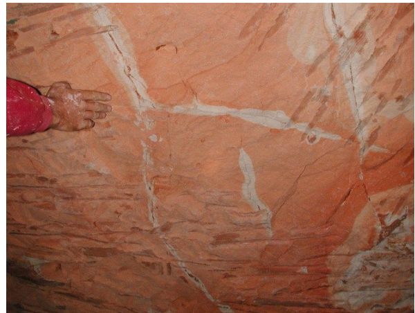
Figure 35 - Joints in a mine roof
