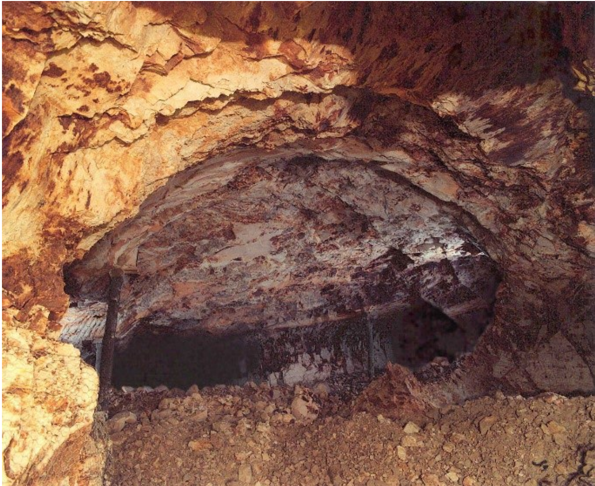
Figure 28 - Arch formation following a roof fall
