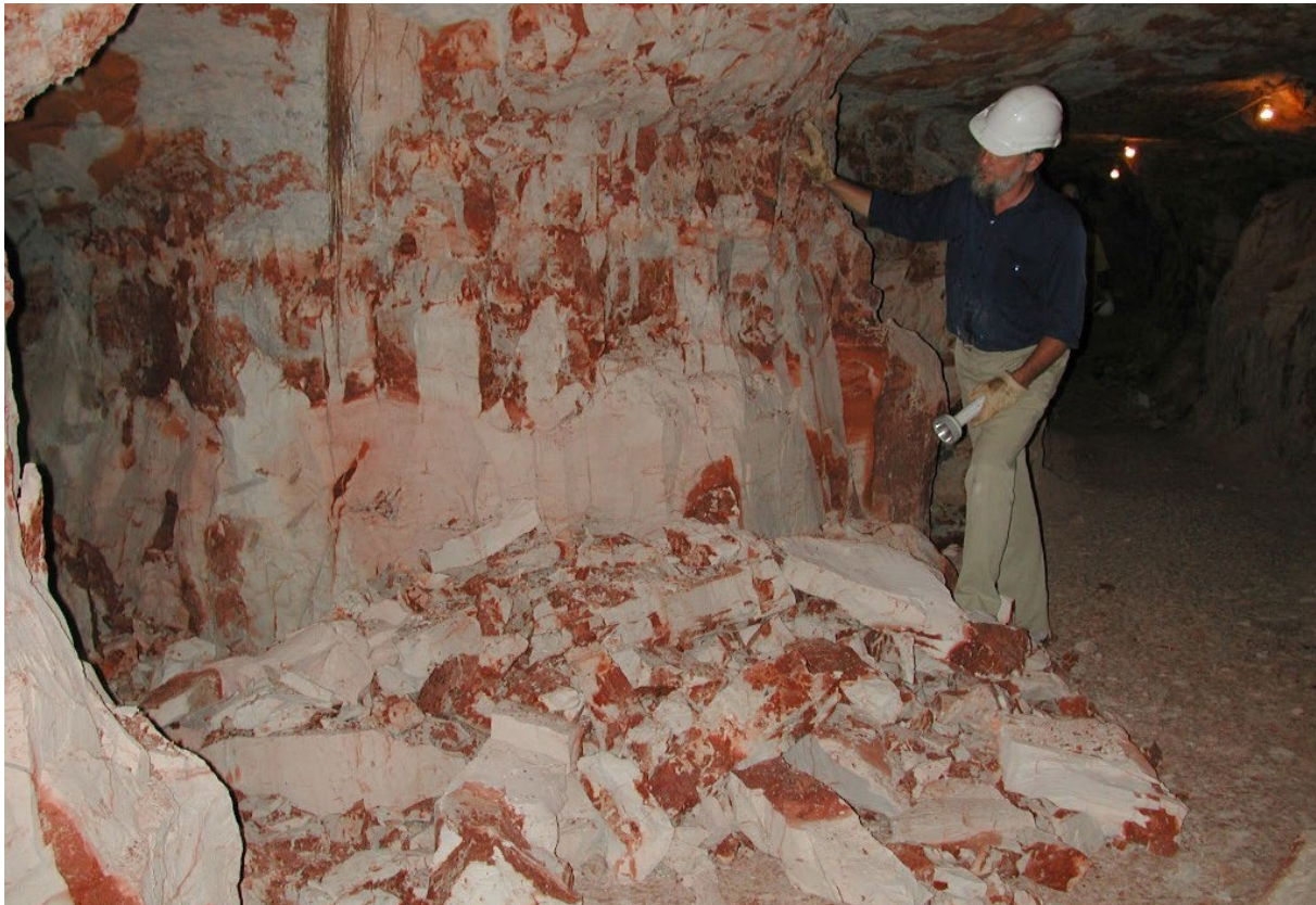
Figure 70 - Fretting pillar
