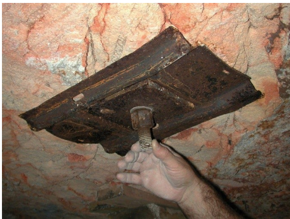
Figure 64 - Rock bolt in roof
