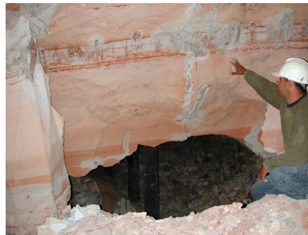
Figure 31 - Bedding planes in roof of a drive
