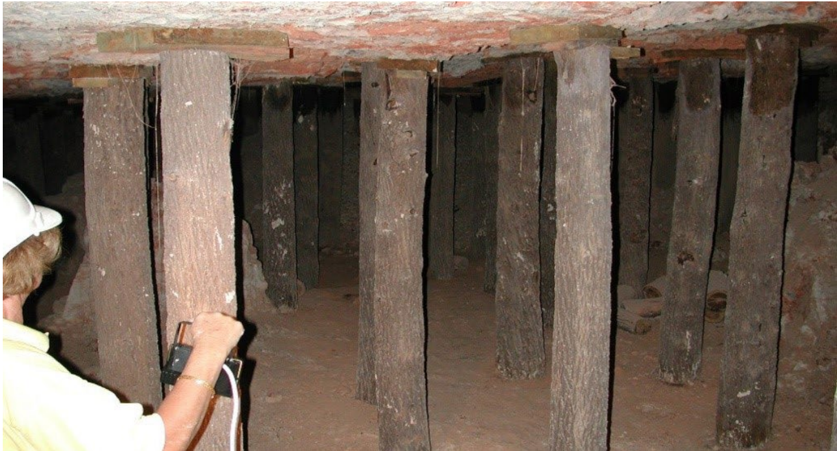
Figure 54 - Planned installation of props
