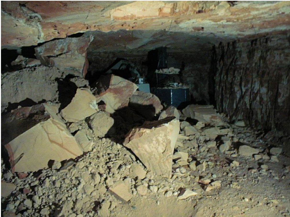
Figure 44 - Large blocks of sandstone that fell from roof resting on mound of backfilled shaft.
