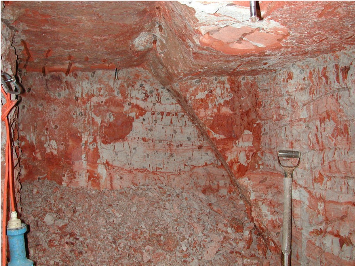
Figure 4 - Example of a fault exposed in a mine drive
