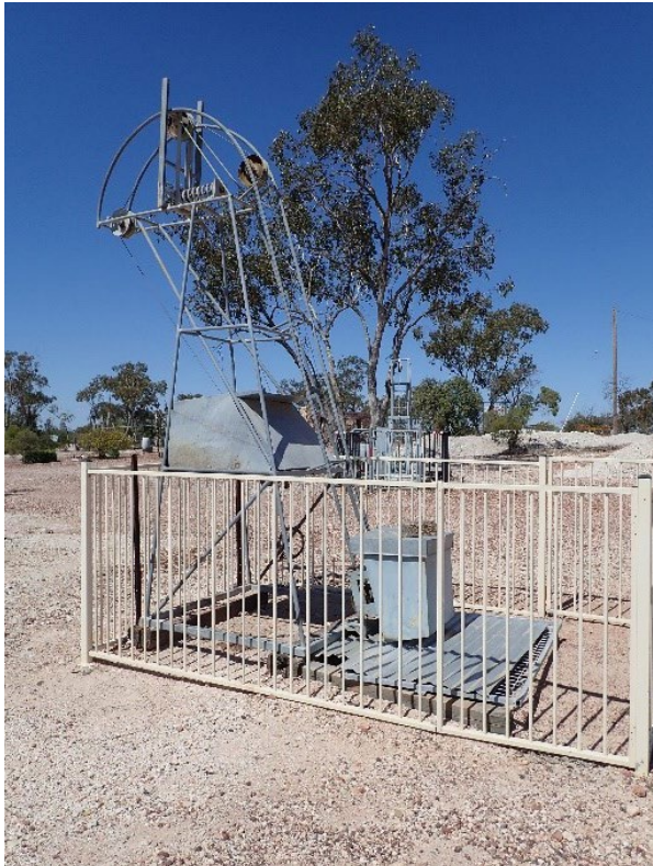
Figure 101 - Opal shafts with both fencing and shaft cover.
