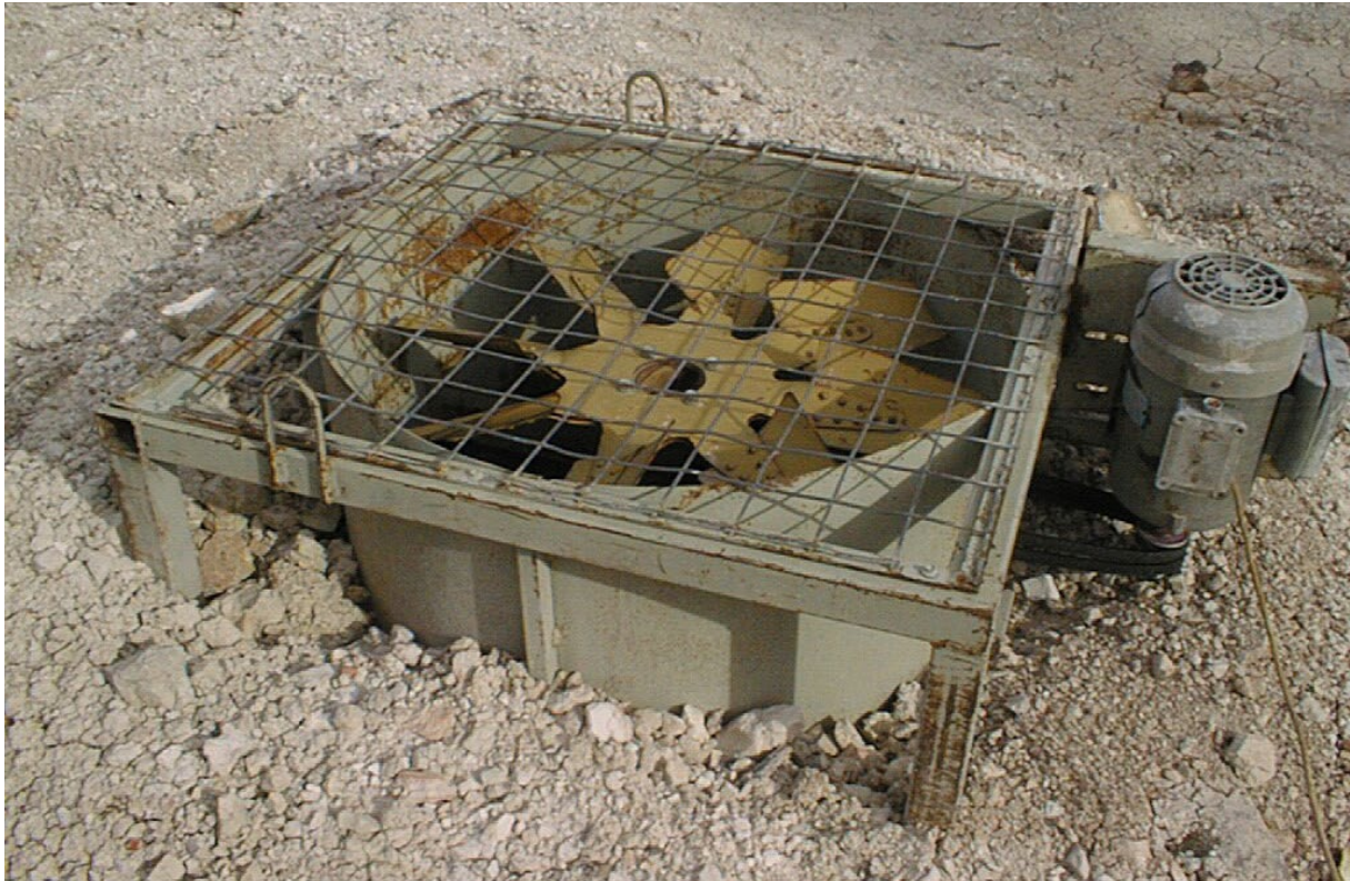
Figure 86 - Electric ventilation fan over a mine shaft
