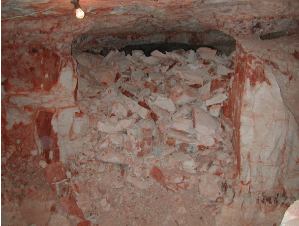
Figure 73 - Backfill supporting pillars
