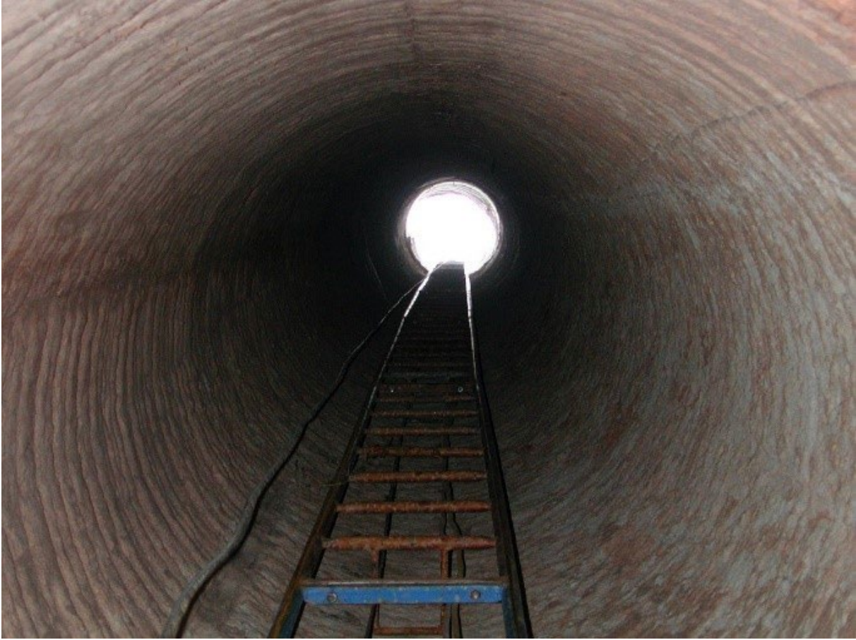
Figure 49 - Rifling effect in a Caldwell hole
