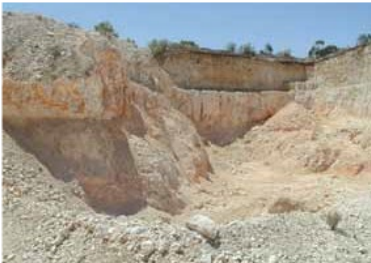
Figure 93 - Benching in the Three Mile open cut at Lightning Ridge
