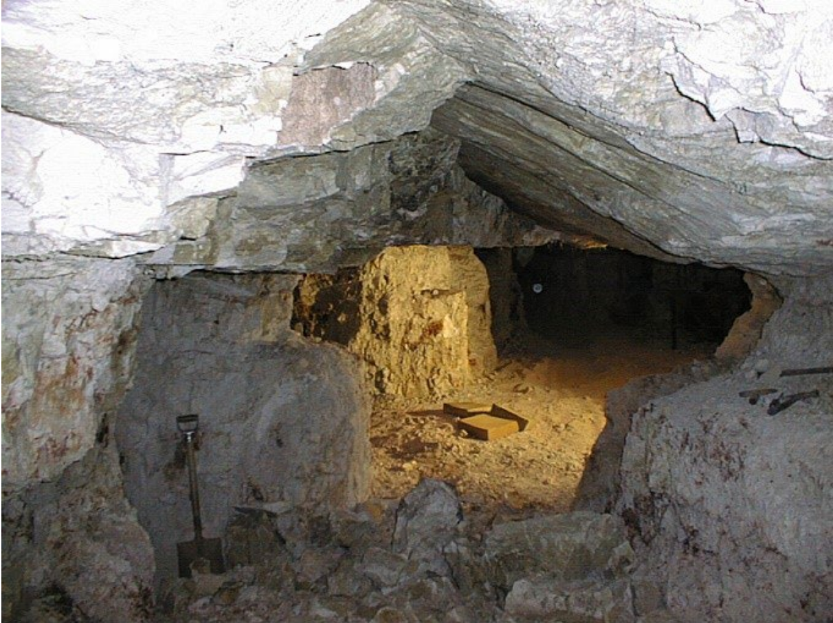
Figure 42 - View of fault plane and fallen rock at Glengarry.
