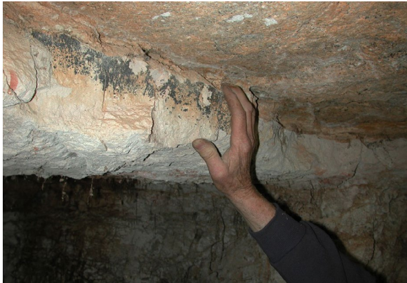
Figure 19 - An example of a loose end - a rock layer that needs to be barred down
