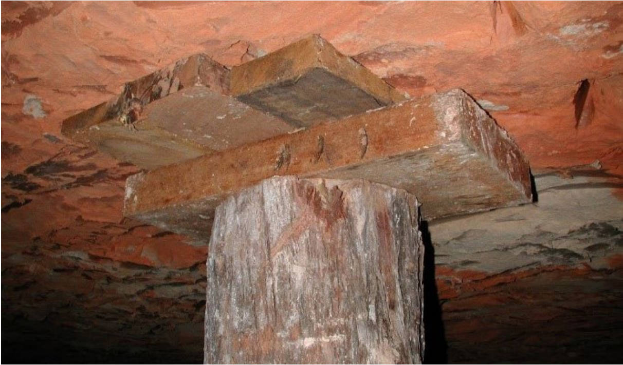
Figure 60 - Wedges filling gap between the mine and the hardwood cap on a prop.
