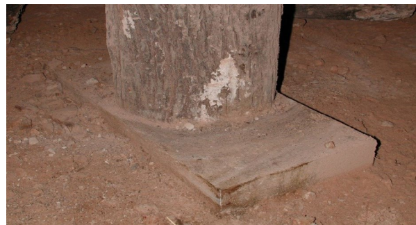
Figure 56 - Props with a base plate
