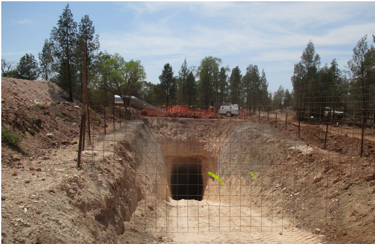
Figure 81 - Underground access using a decline
