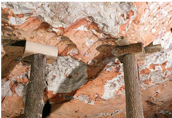
Figure 55 - Props with a softwood cap
