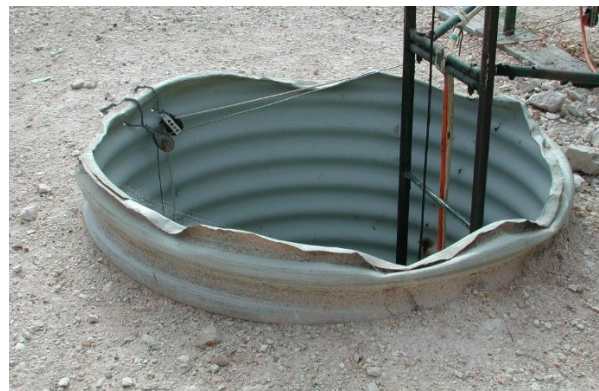
Figure 12 - Collar protected by galvanised iron
