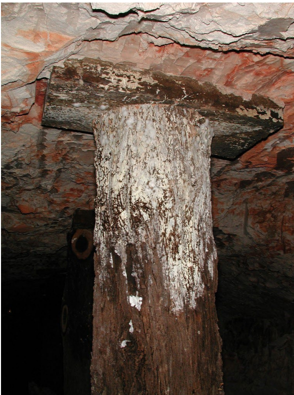
Figure 62 - Initial stages of fungus growth on a prop.
