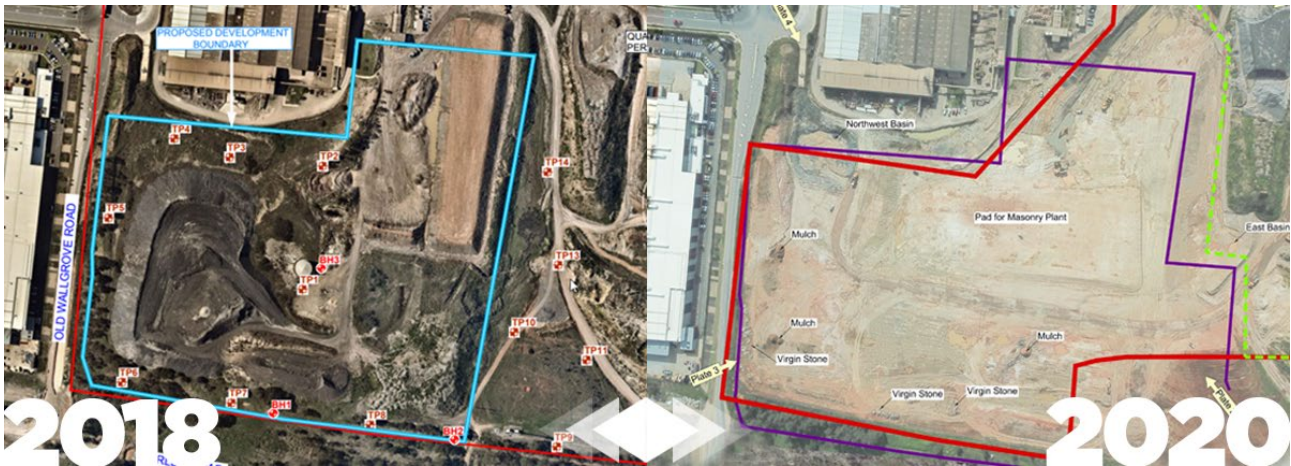
FIGURE 1. REHABILITATION AT THE HORLSEY PARK QUARRY SITE
