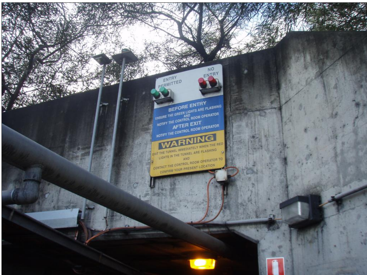
Figure 9. Entrance to reclaim tunnel.
