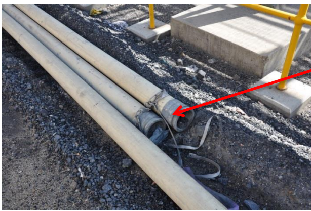
Figure 15 – Recovered poly pipes towed out of the mine.
