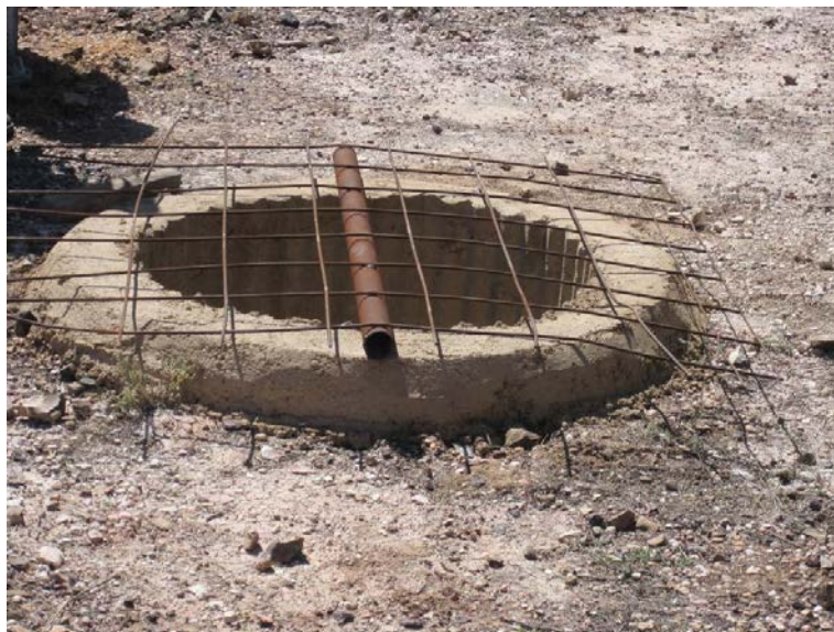
Figure 7 The shaft showing the steel mesh in what was alleged to be its usual position on 7 March 2013. Note that the mesh was placed over the shaft after the incident.
