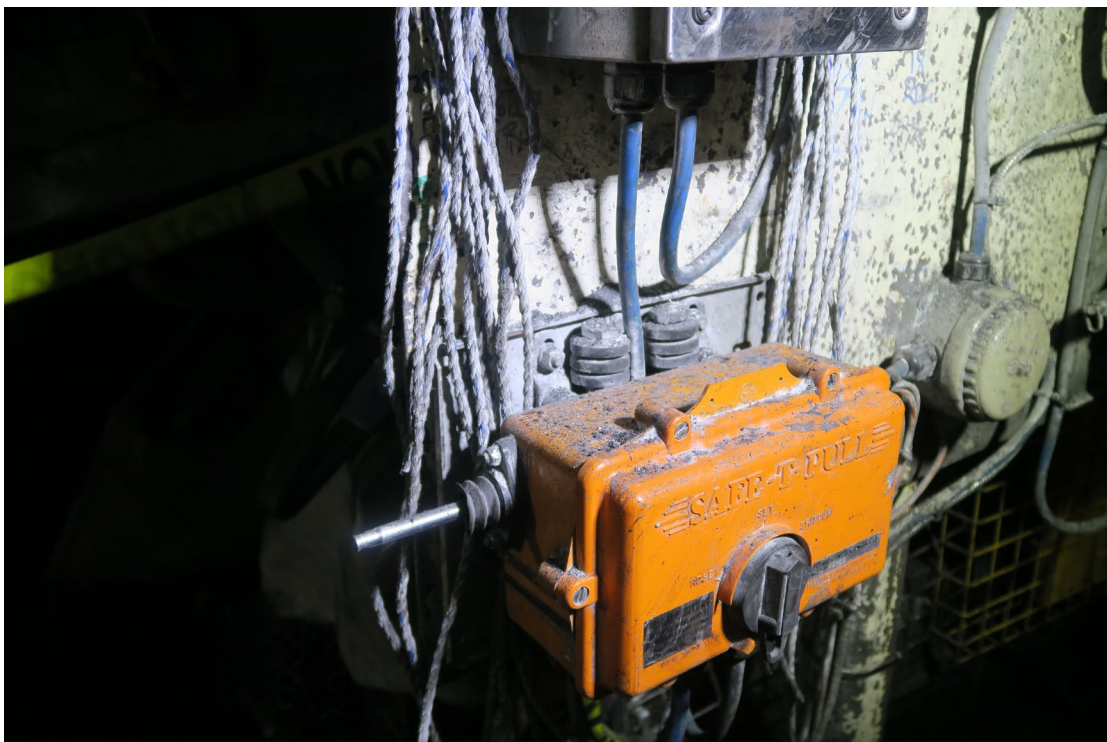
Figure 15. Emergency lanyard control box with missing lanyard
