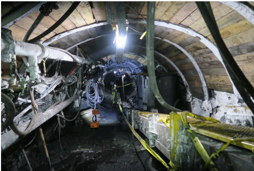
Figure 3. The new scraper conveyor at Appin North post incident
