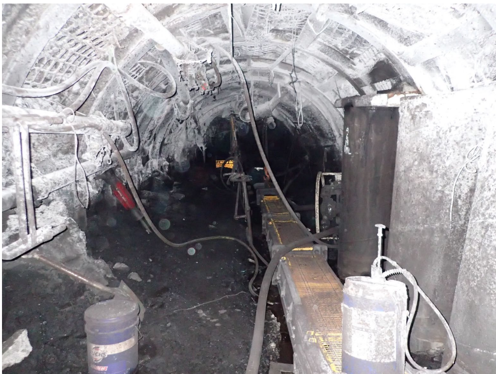
Figure 7. Walkway covered in material
