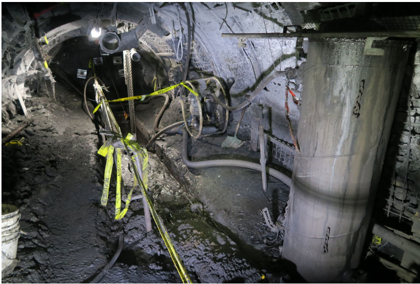
Figure 4. Concrete sump at Appin North (scraper conveyor pick up area)
