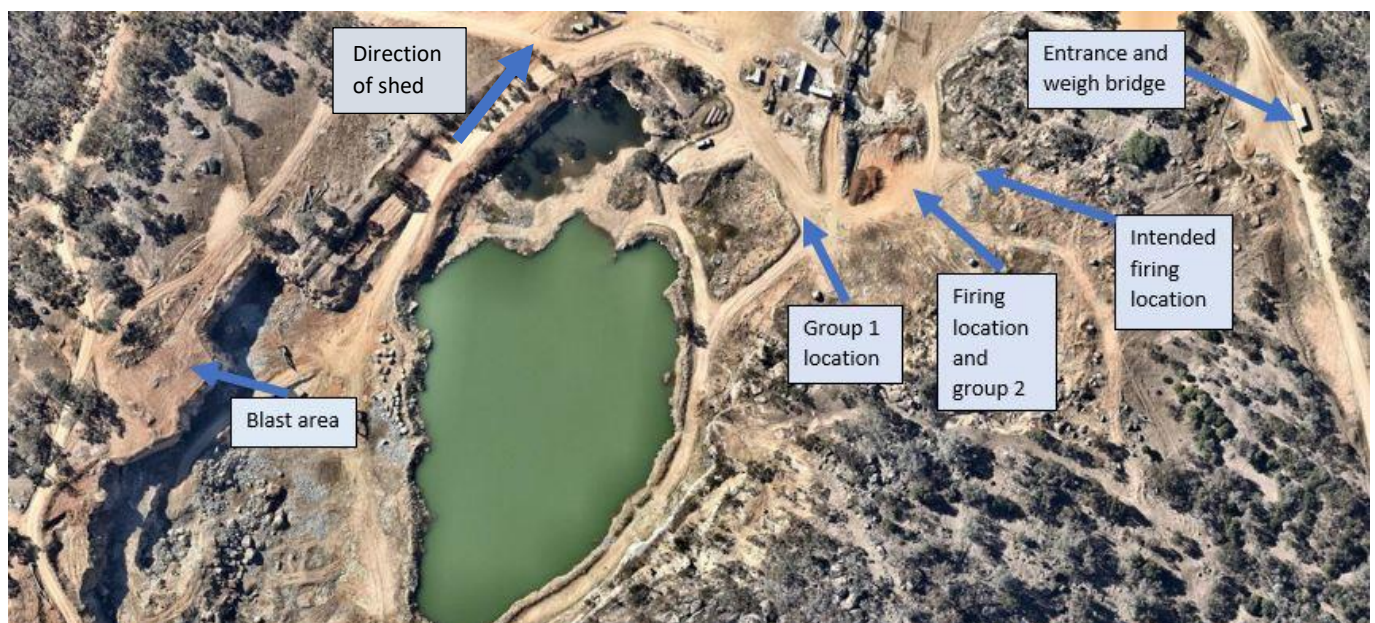
Figure 6 - Key locations at quarry
