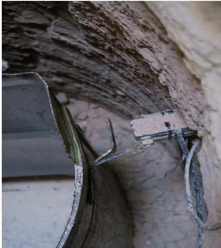
Figure 11: The bucket in the sump (bracket and limit switch).
