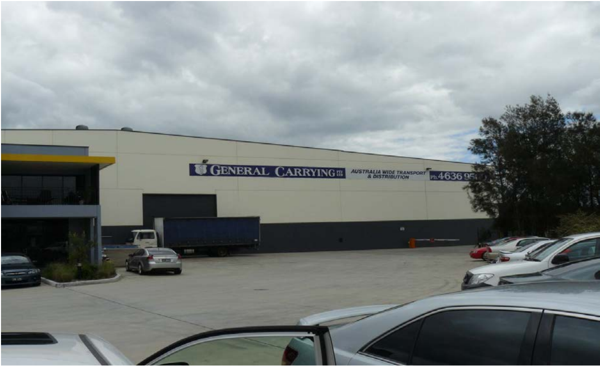
Figure 4: General Carrying's warehouse at Smeaton Grange on 14 December 2011.
