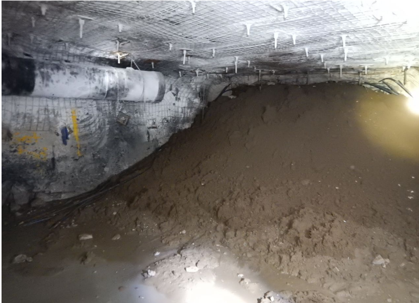
Figure 2: Bulkhead seal failure
