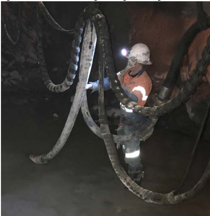
Figure 1 A worker simulating clearing a blockage in a shotcrete delivery line
