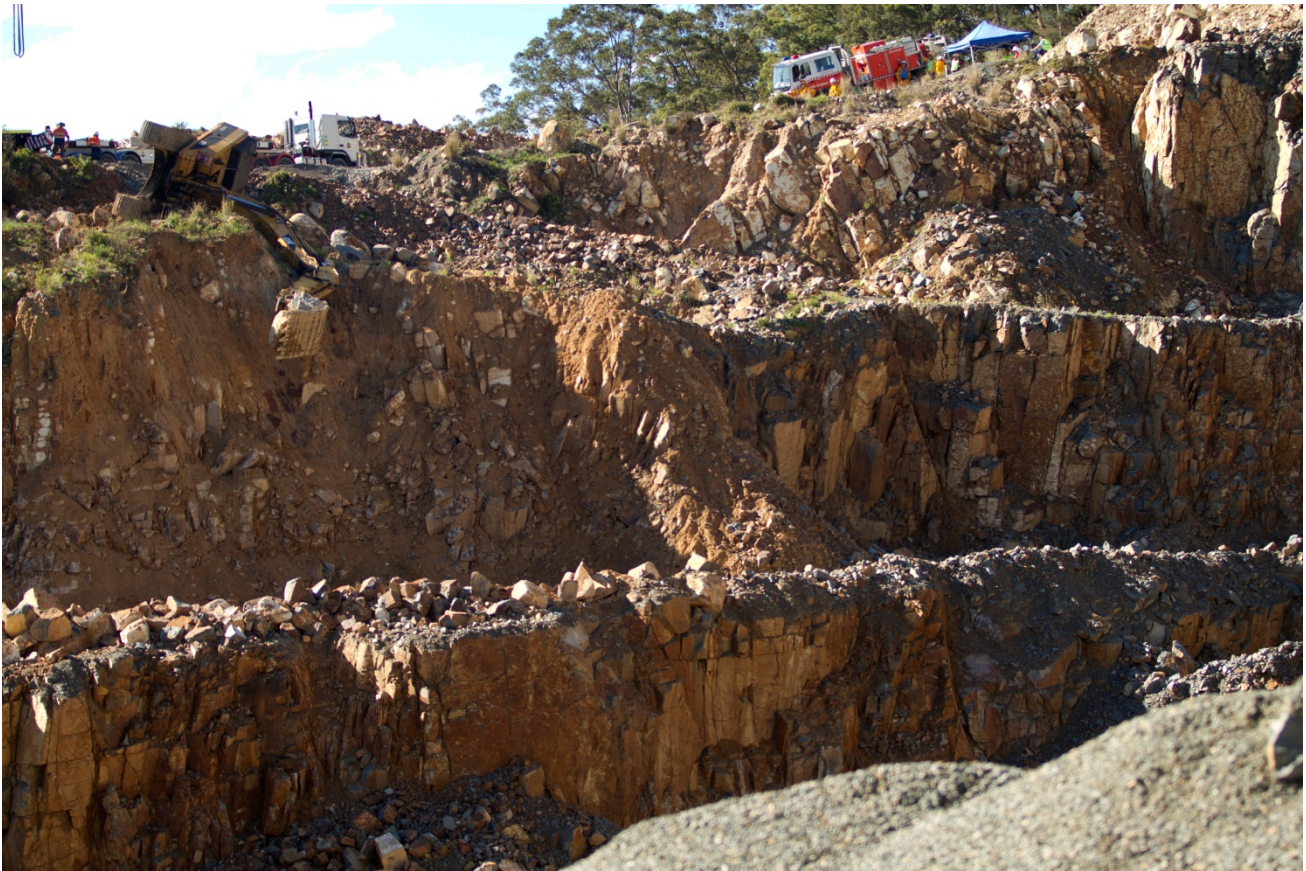
Image 2: Bench and quarry face –showing rock in excavator bucket - Photograph by Investigation Unit
