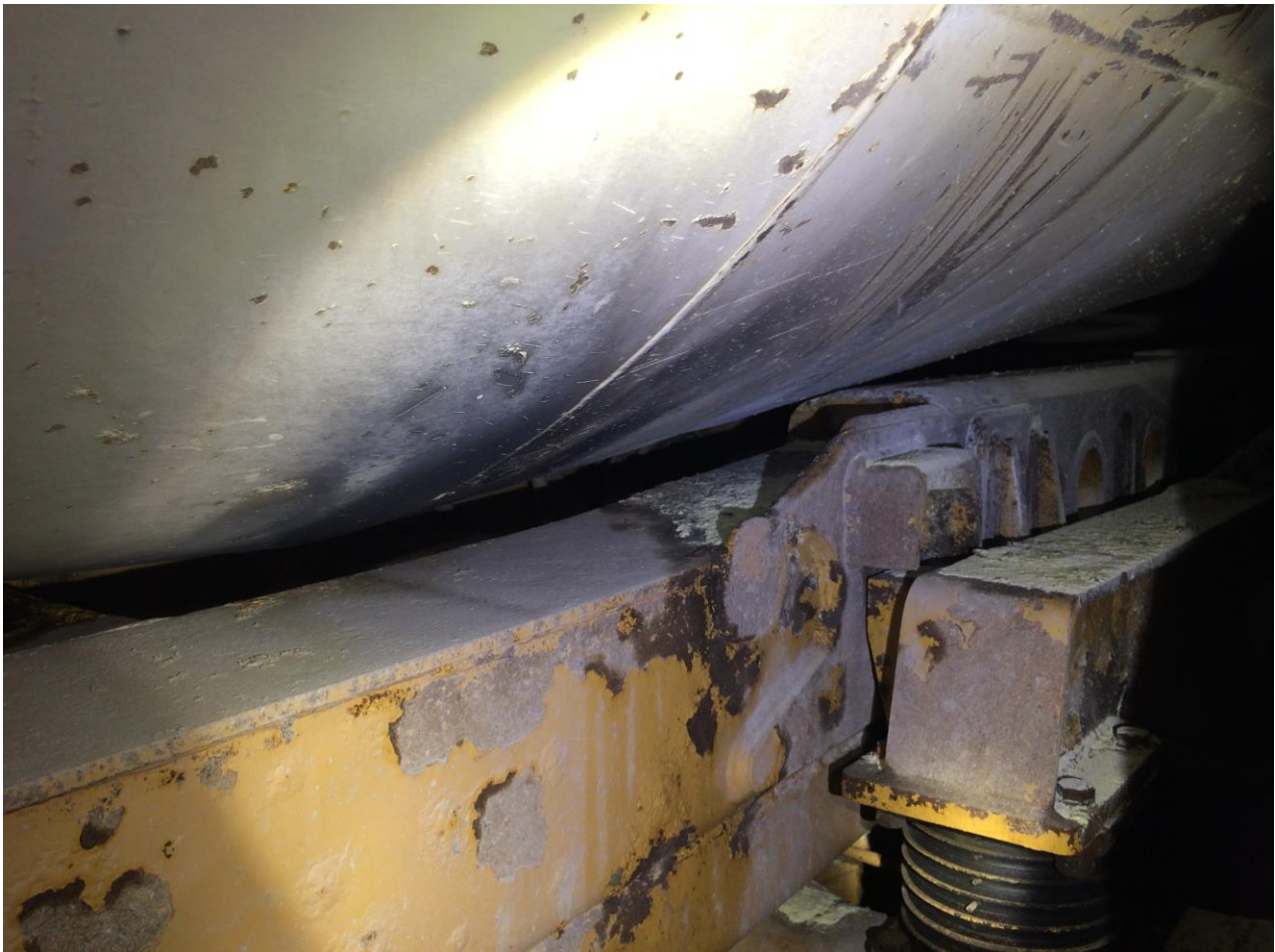
Figure 20. Cadia East underground
