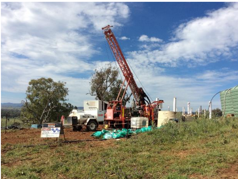
Figure 7 Drilling rig at site 20JNDD001
