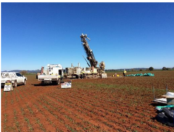
Figure 4 Durock Drilling rig on site at 20LIRC010
