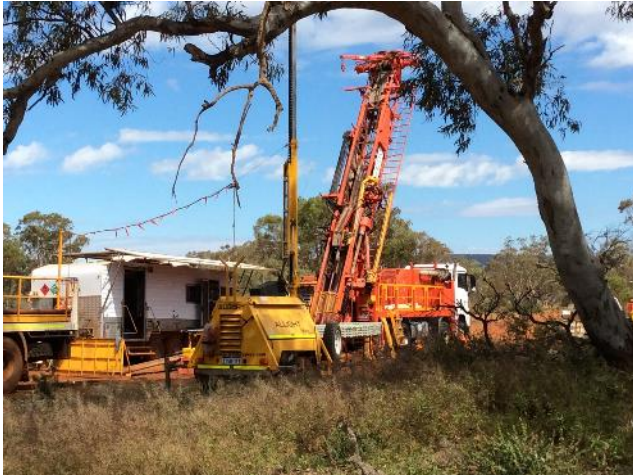
Figure 7 Drilling rig at WTRCDD194
