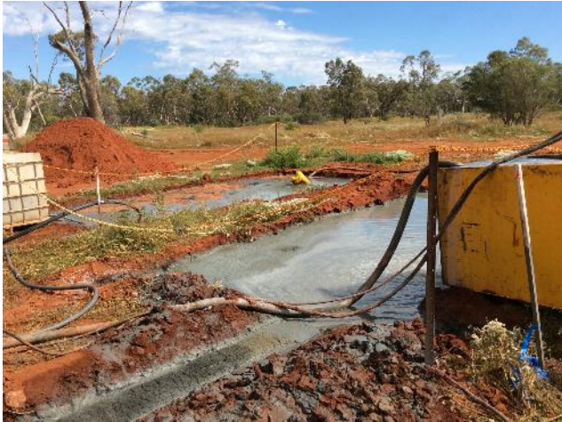
Figure 5 Inground sumps at WTRCDD194
