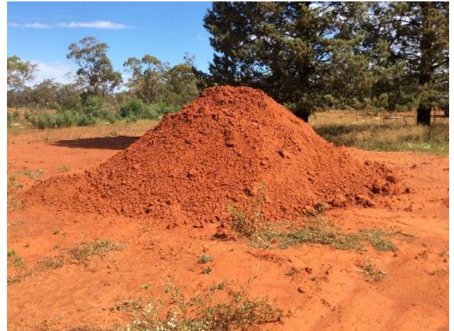
Figure 8 Topsoil from sump excavation stockpiled at WTRC195
