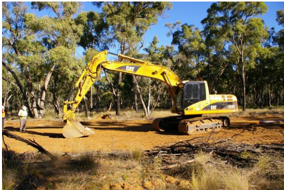
The Cat 320C excavator at the incident scene.
