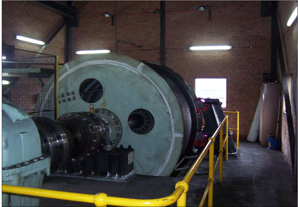
Single rope drift winder drum
