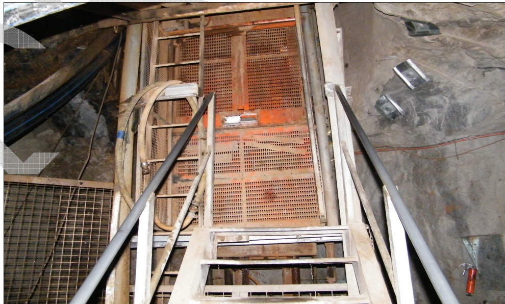
Raise climbing winder conveyance with trailing cable
