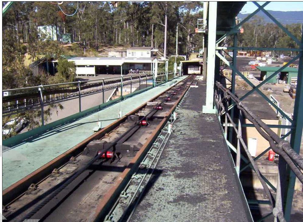
Single rope drift winder conveyance entering a drift
