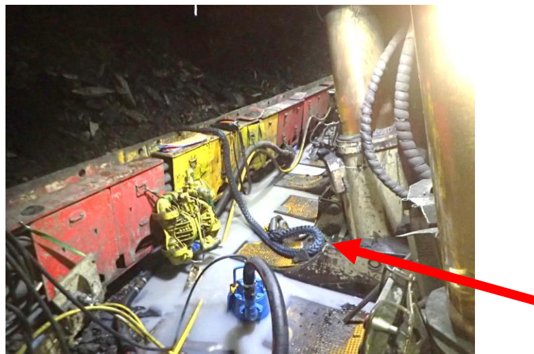
Figure 1: Location of worker struck by the recoiling shackle and blue Amsteel® rope
