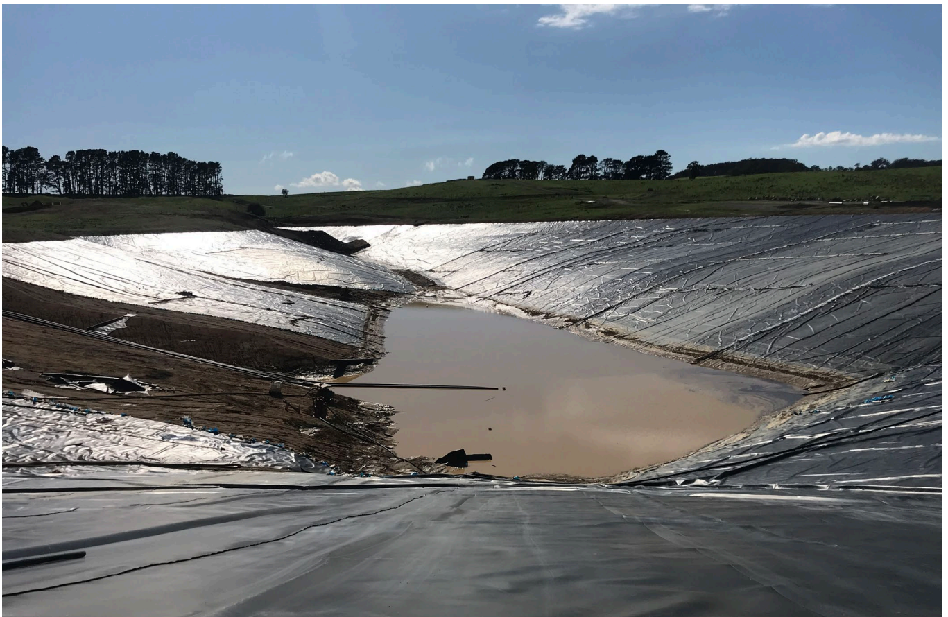
Figure 2 Lined tailings storage facility under construction in southern NSW
