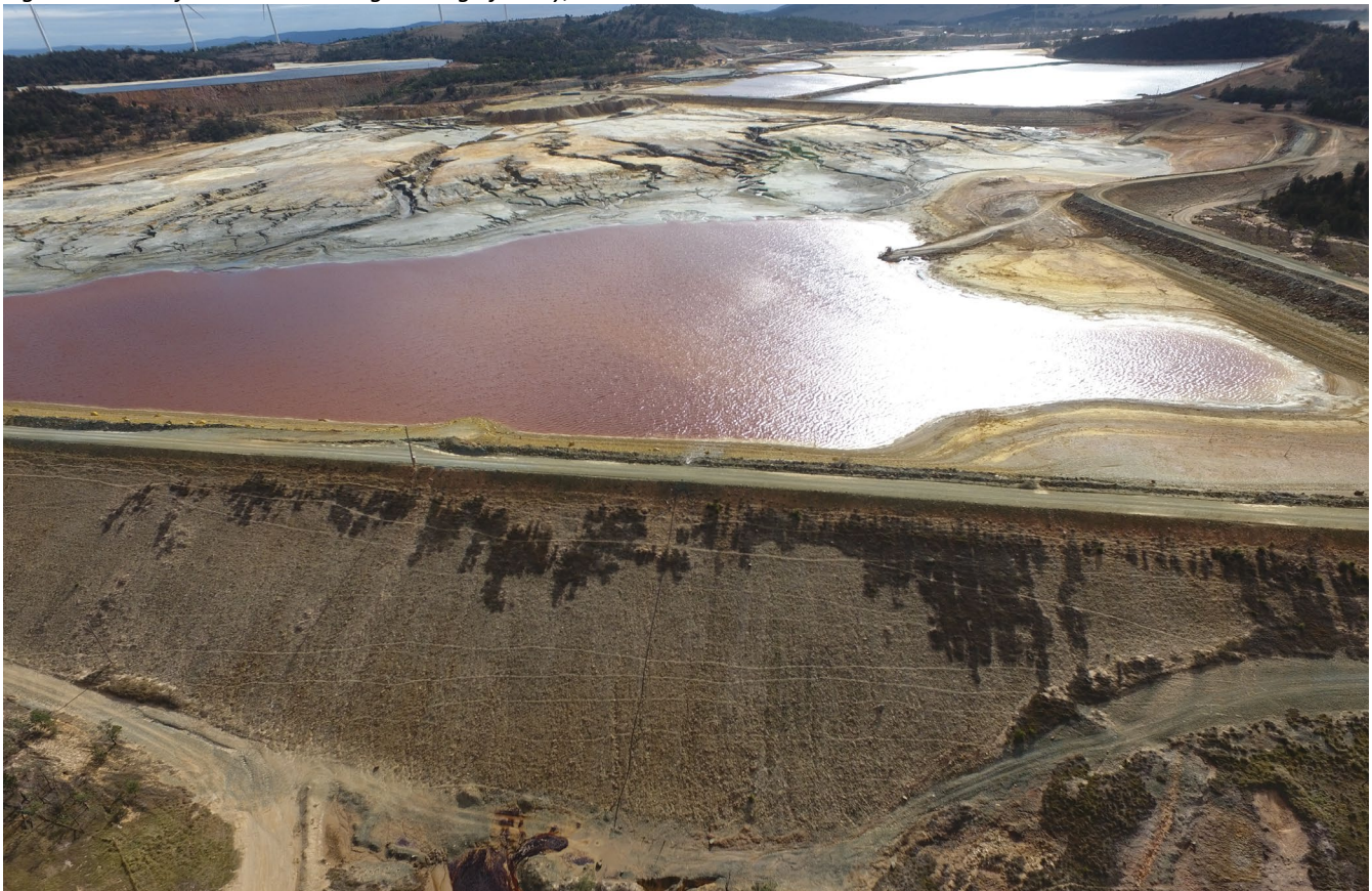
Figure 1 Metalliferous mine tailings storage facility, southern NSW
