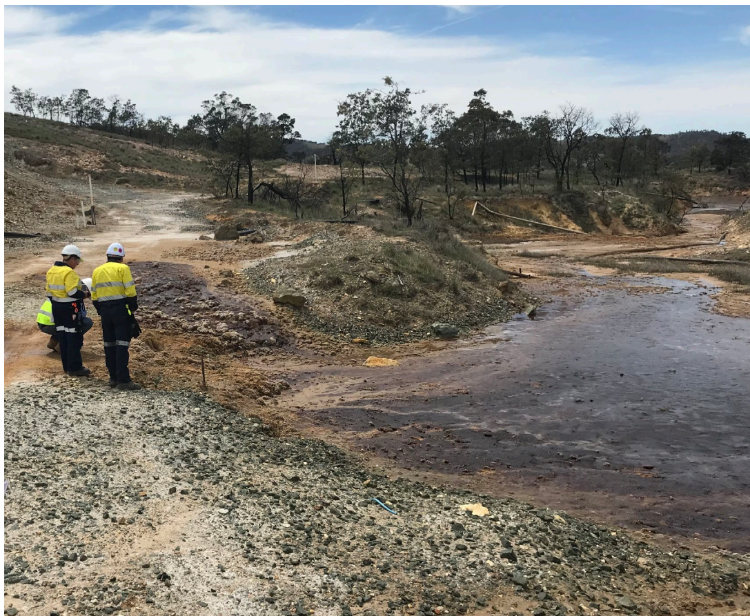
Figure 3 Government inspectors assessing tailings dam seepage
