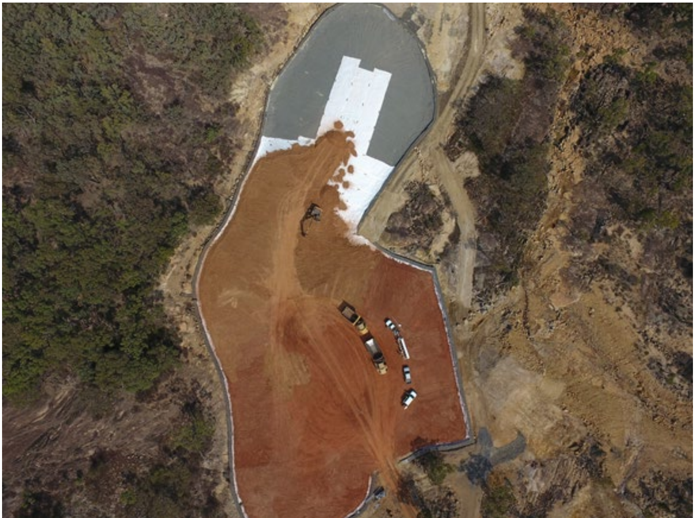
Figure 8 Placement of an engineered cap on legacy tailings facility - northern NSW
