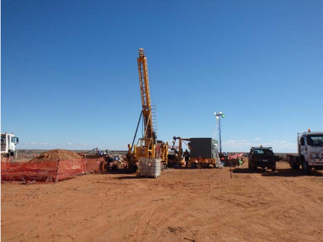
Figure 9 Drill site marked with flagging tape and barrier fencing
