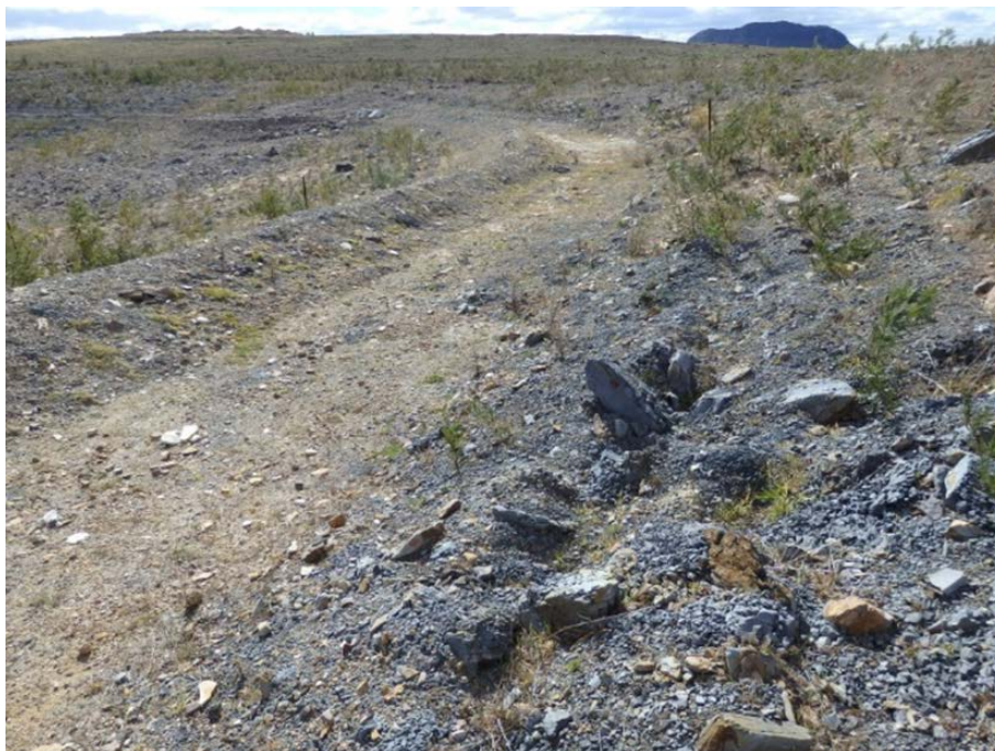
Figure 2 Contour berm at Stony Creek rehabilitation, protecting a slope from erosion
