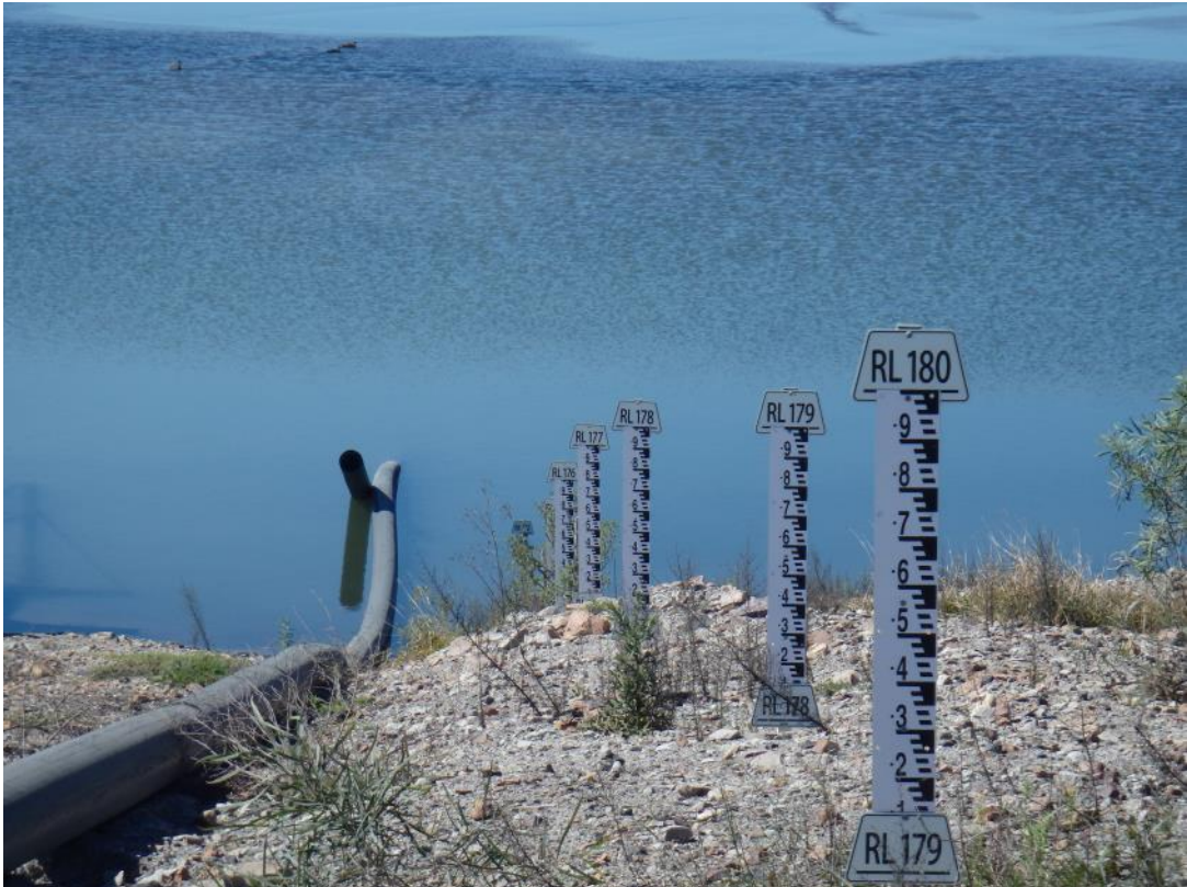
Photo 13 – Example of manually read gauge marker boards in a tailings dam
