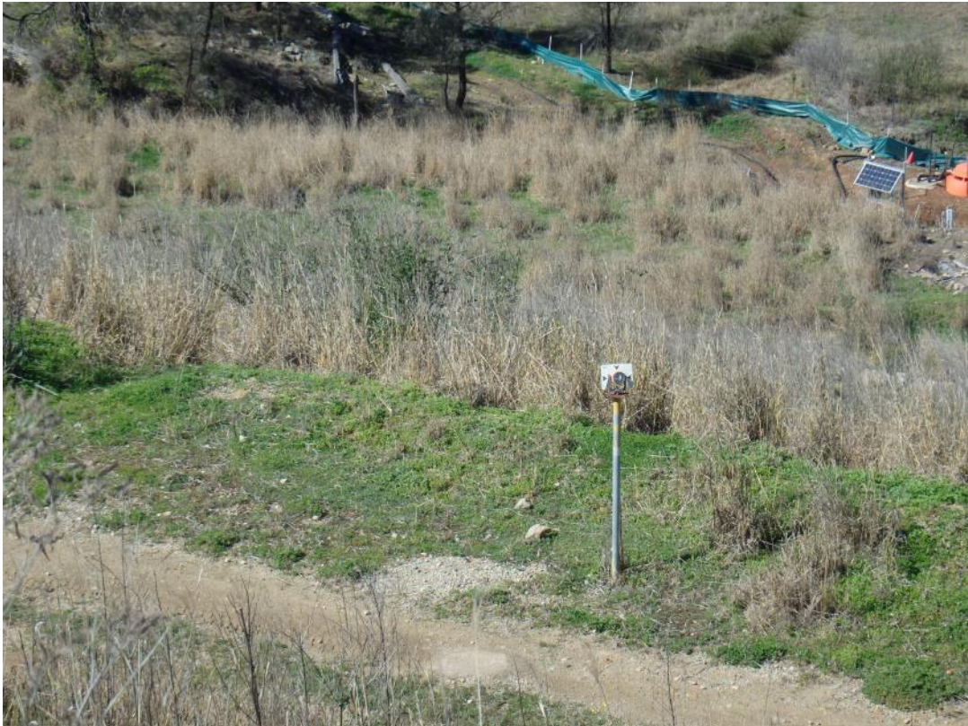
Photo 11 – Example of movement survey prism on a dam embankment
