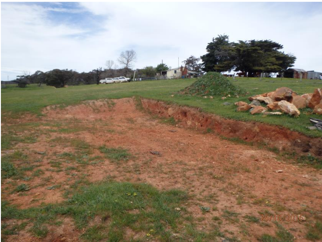
Photo 6 – Unrehabilitated drill site – drilling was completed in early 2016
