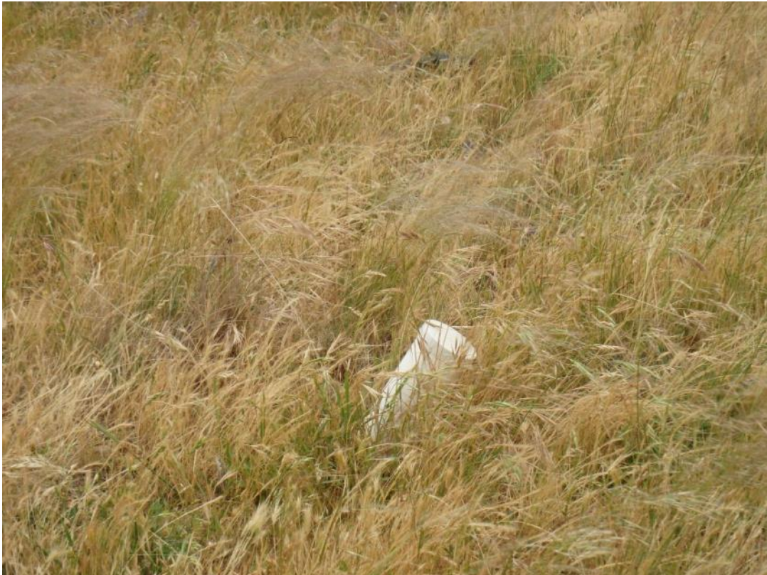
Photo 1 – Casing protruding from the ground on a rehabilitated borehole site
