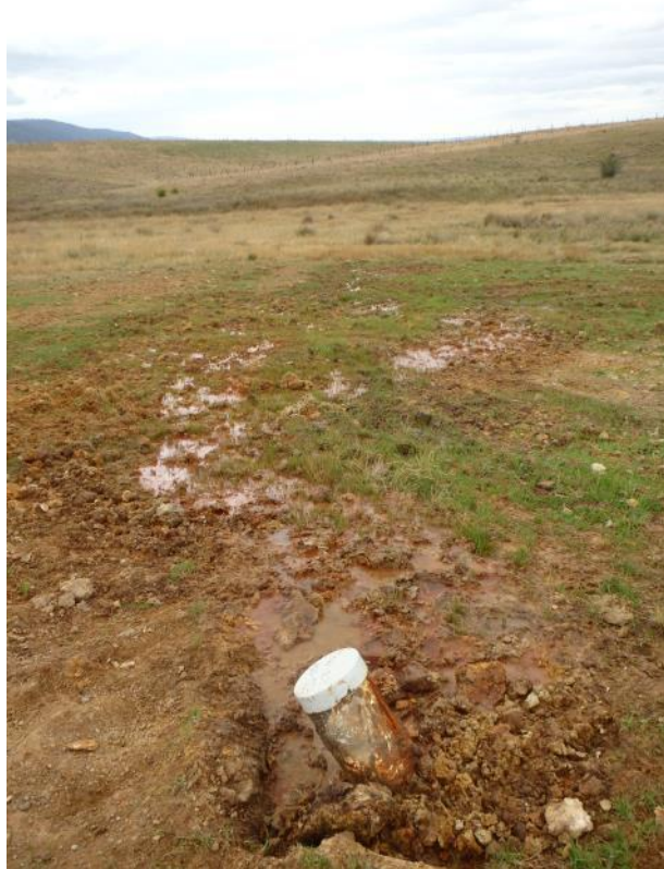
Photo 5 – Groundwater leaking from a borehole
