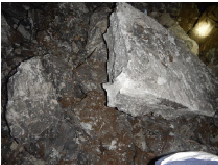
Figure 5 Failed cementitious product recovered from the failed bulkhead
