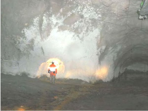
Photograph of ventilation wall at intersection near top of VR5B shaft – 760m from base of VR5A shaft.
