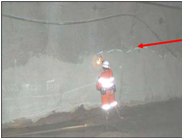
Photograph near base of VR5A shaft.
