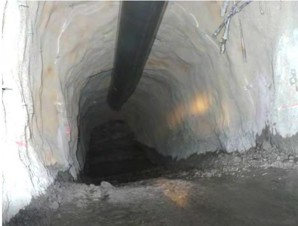
Photograph of sump at bottom of decline.
