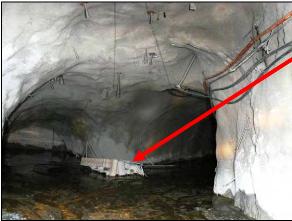
Photograph of the mini excavator that was washed approximately 300 metres along the drive to top of VR5B shaft.
