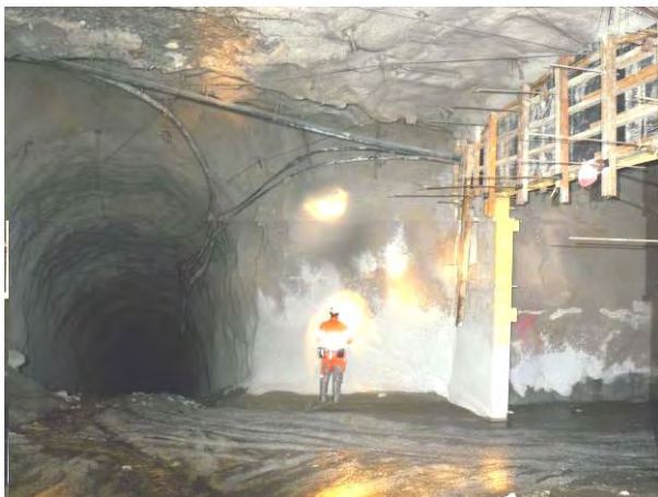
Photograph of roadway intersection 550m from base of VR5A shaft.
