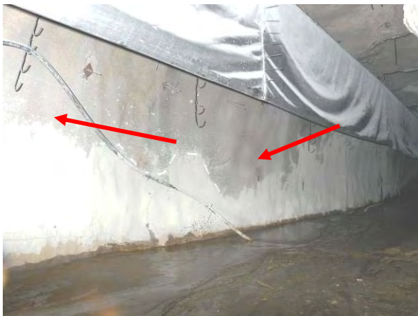
Photograph at base of VR5A shaft.
