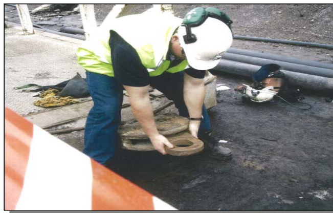
Photo showing re-enactment of lifting the cassette coupling
