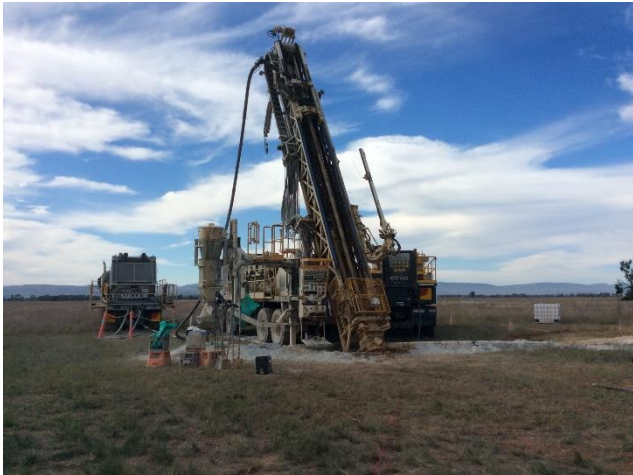
Figure 1 Strike Drilling RC rig set up at site EPP042
