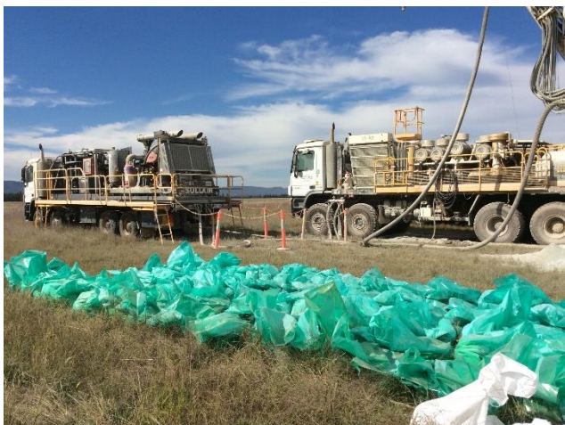
Figure 8 Strike Drilling rig in cleared paddock
