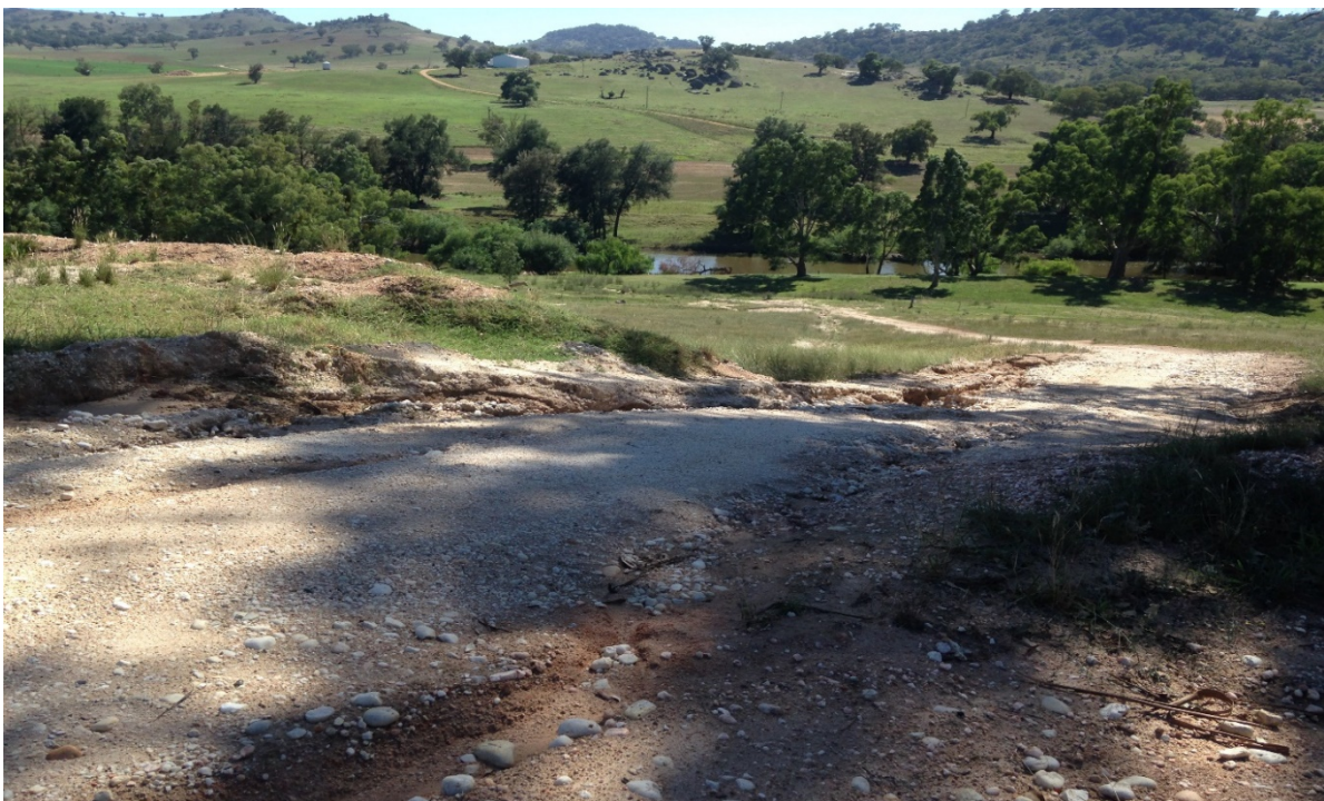
Figure 8 Erosion on road on northern edge of disturbed area (facing north)
