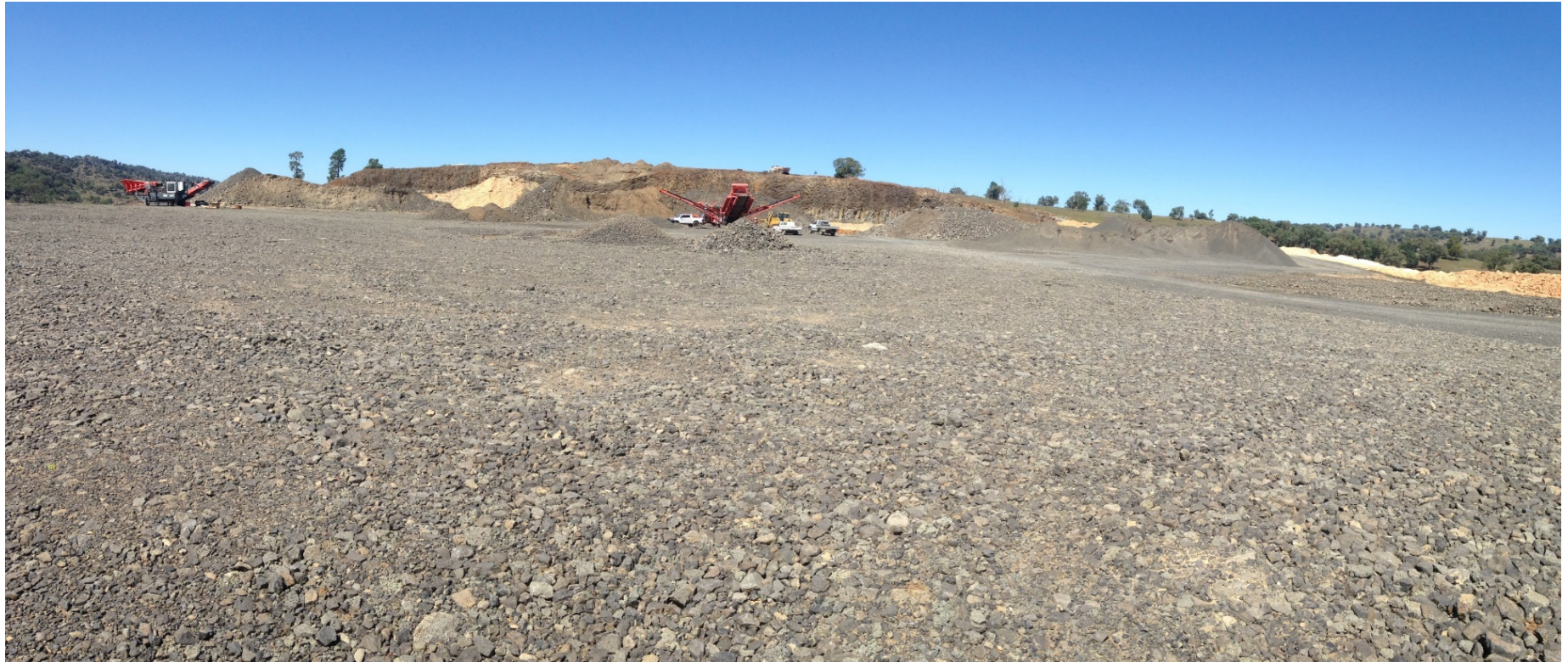
Figure 9 Progressive backfill on quarry floor
