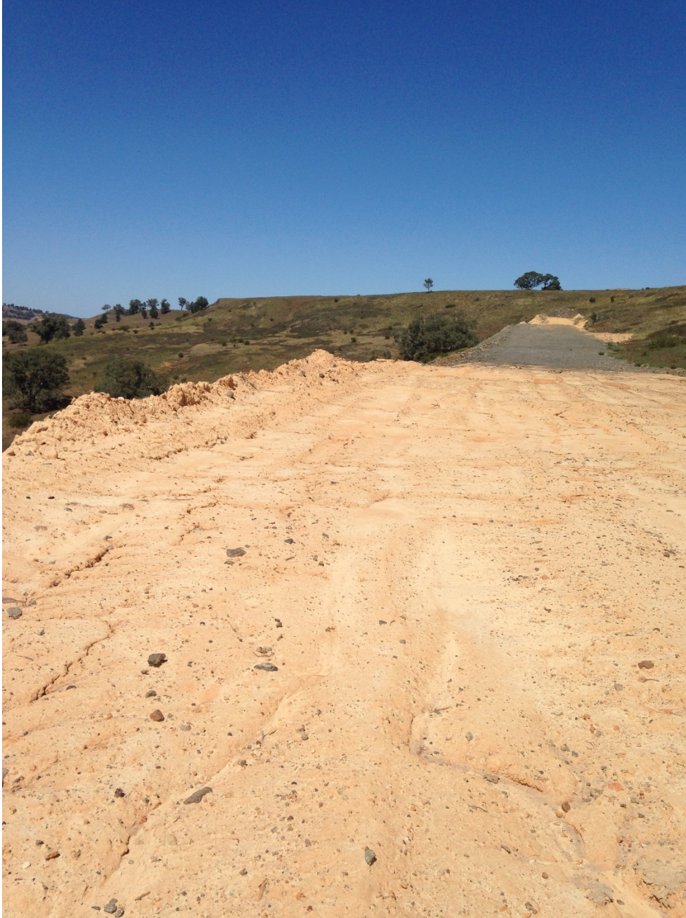
Figure 12 New exit road on eastern side of operation (facing south)
