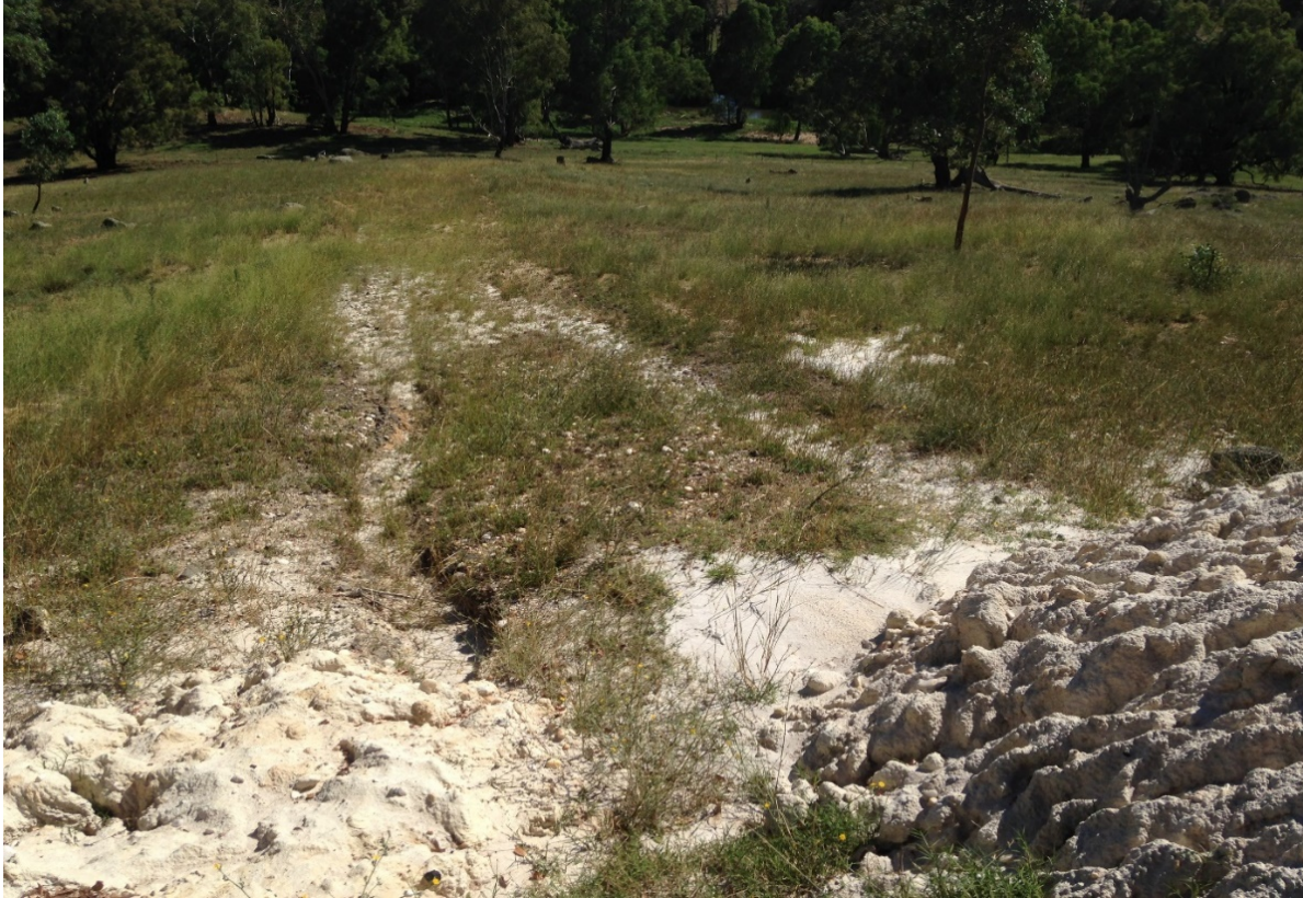
Figure 8 Erosion on road on northern edge of disturbed area (facing north)
