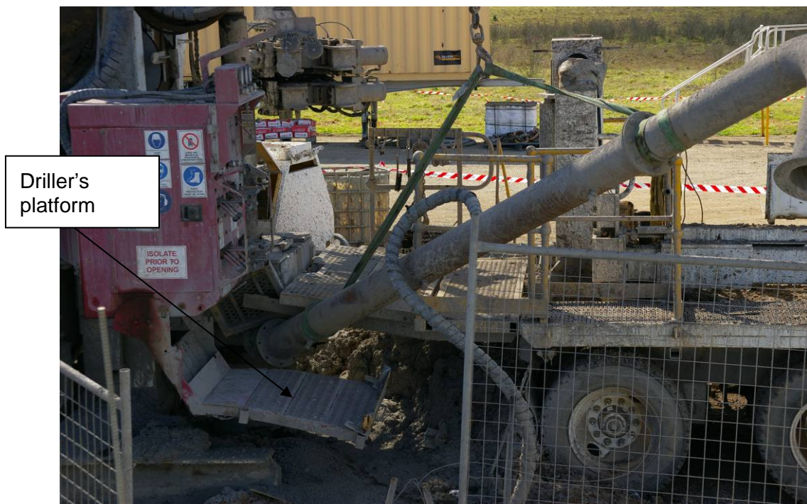
Figure 8. Drilling platform and elevated air discharge line.
