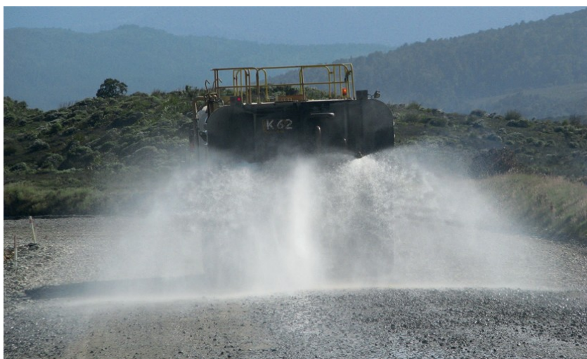
Figure 4: Dust suppression using a mobile tanker.
