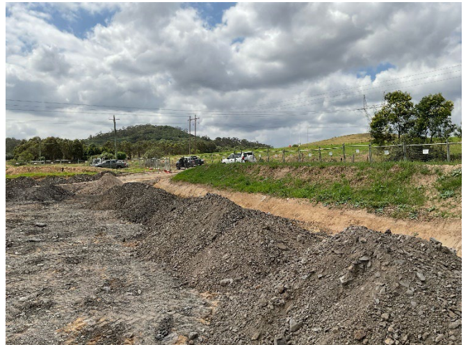
Figure 8: Well sites MP16 and MP25 - rehabilitation in progress using a rural pasture rehabilitation model
