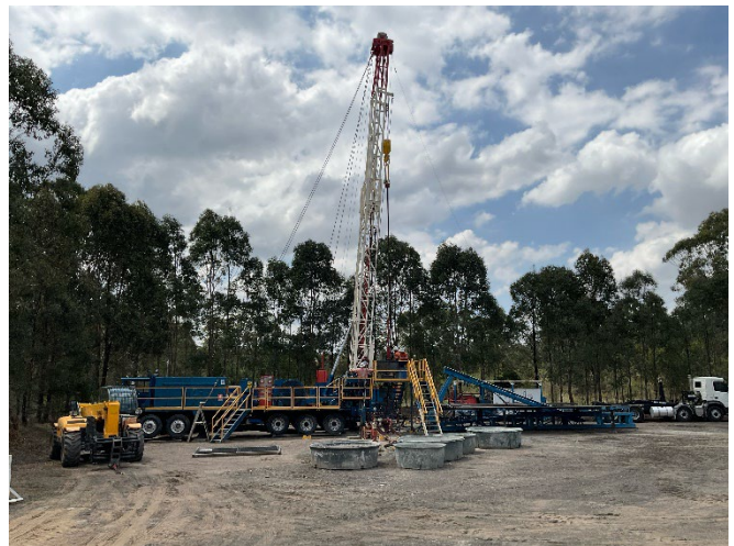
Figure 4: Workover rig on well site Sugarloaf 7 - plugging and decommissioning in progress
