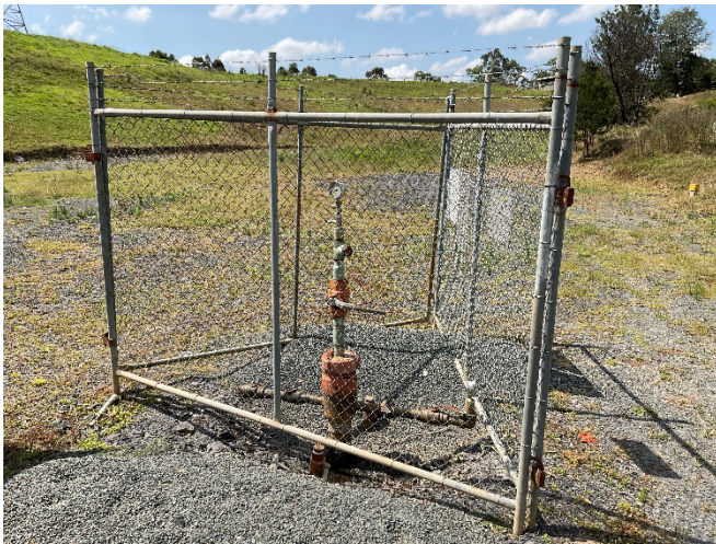
Figure 3: Wells Menangle Park 1, 2, 3 and 9 - all wells plugged and decommissioned awaiting cut and cap
