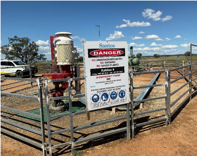
Figure 3: Stock fencing around the Kahlua 4 well site
