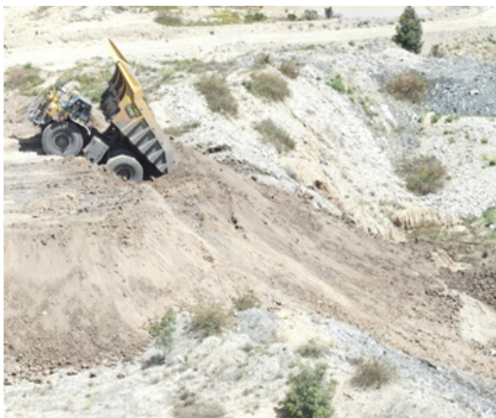
Picture 13. Slumped material and truck
