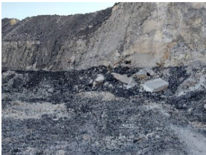
Picture 3. Highwall rockfall which contacted dozer.
