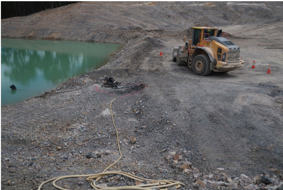
Figure 2: The outlet hose, water pump and dam
