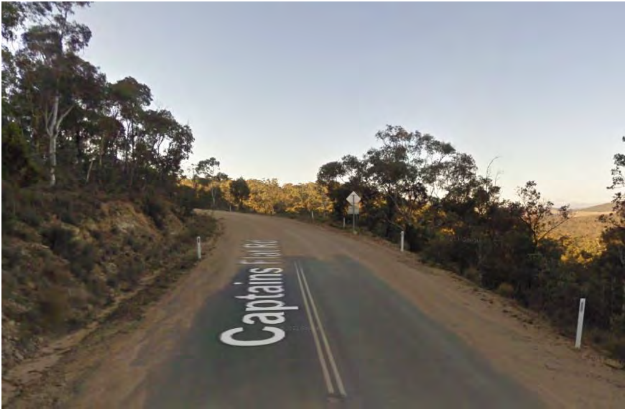
Figure 2: Interface between sealed and unsealed sections of Captains Flat Road located on the southern approach to Captains Flat.
