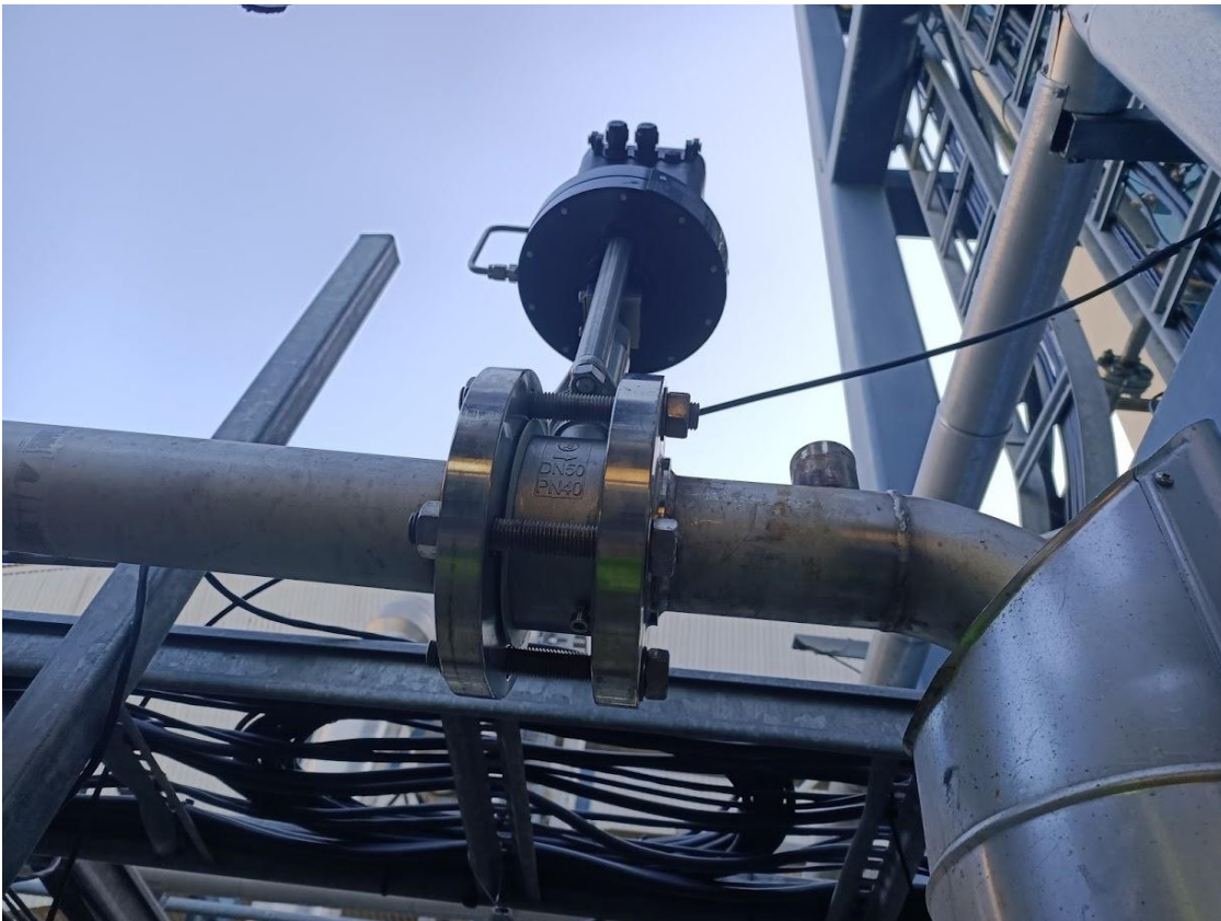
Figure 35 New steam valve installed
