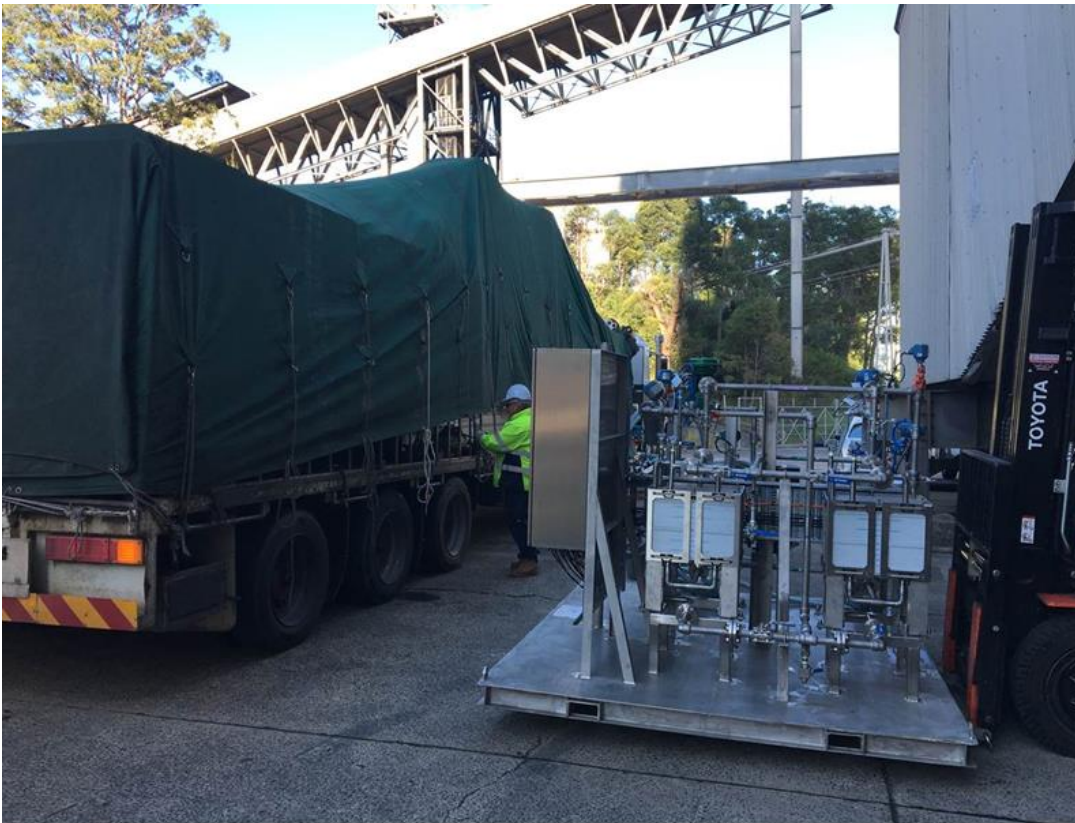
Figure 49 Forward Osmosis unit delivered on site (with 2 membrane modules installed)
