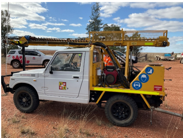
Figure 1 Small vehicle mounted auger drill rig
