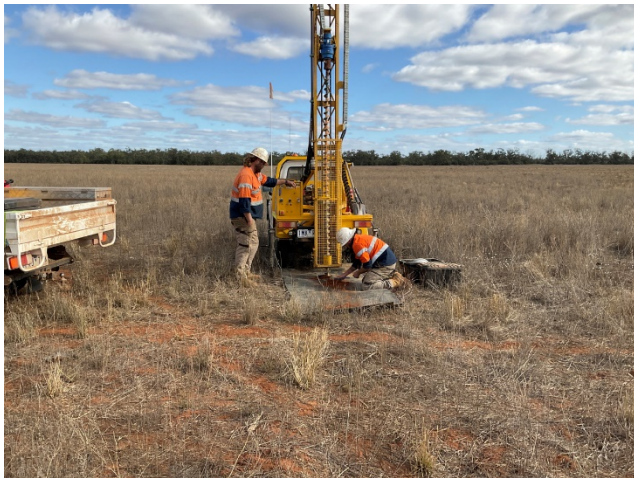
Figure 3 Auger drilling in progress showing minimal site disturbance
