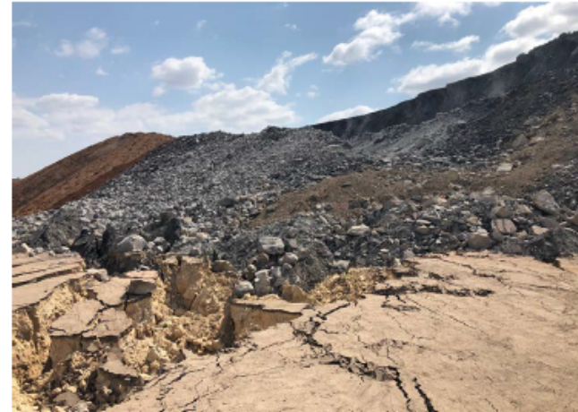
Figure 2 Recent highwall failure January 2020
