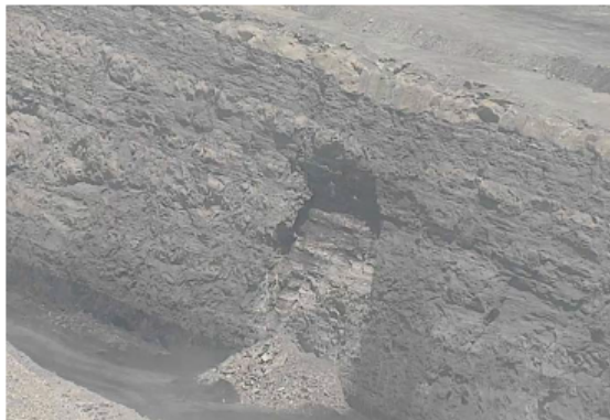
Figure 1 Recent highwall failure February 2020
