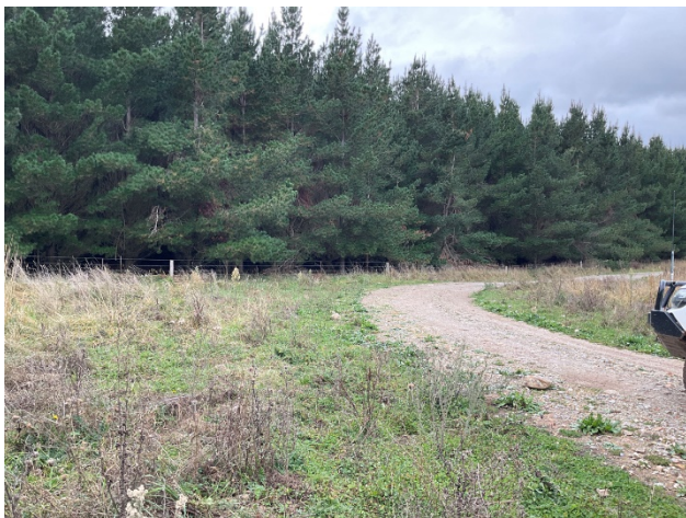
Figure 4 Roadbase on a forestry road to maintain all weather access
