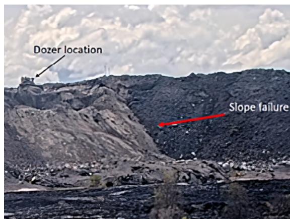
Picture 1. Slump location.
