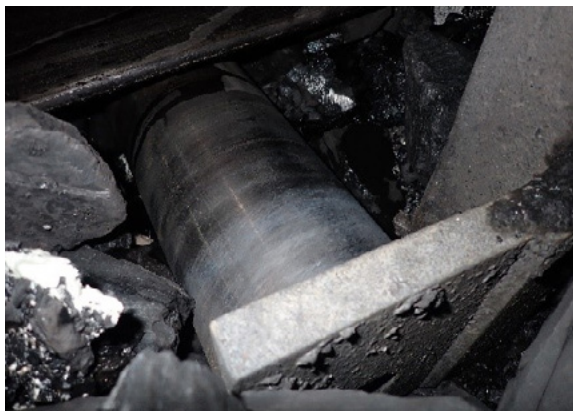
Picture 18. Result of boot end fire.
