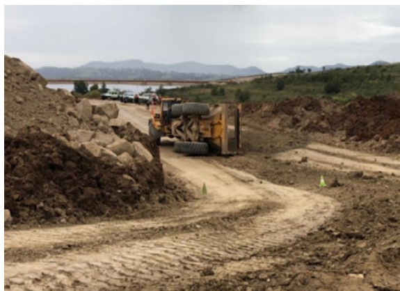
Picture 12. Trailer rollover with cab remaining upright.
