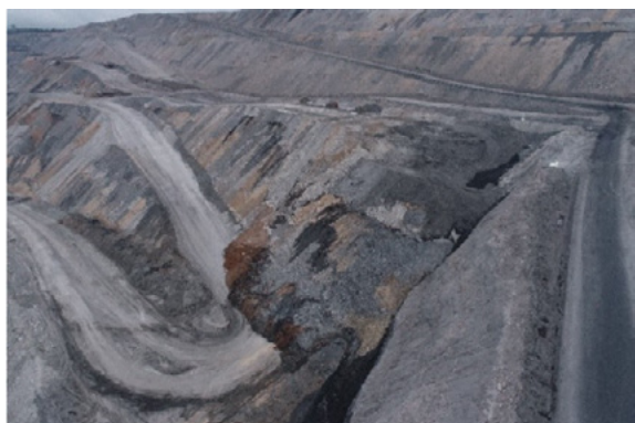
Picture 4. Slump location.
